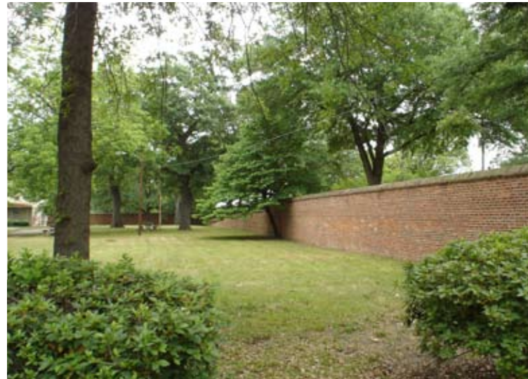
22. Brick wall located along Calhoun Street
