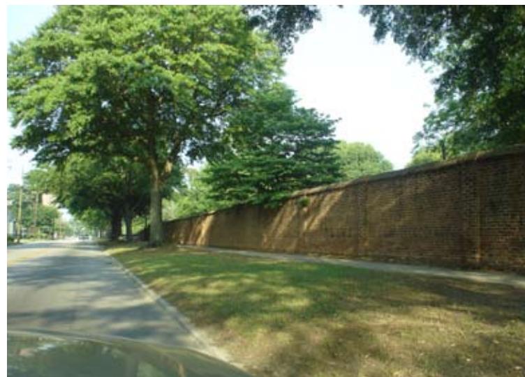
25. Brick wall located along Calhoun Street
