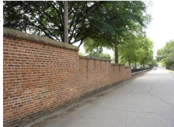
23. Brick wall located along Calhoun Street
