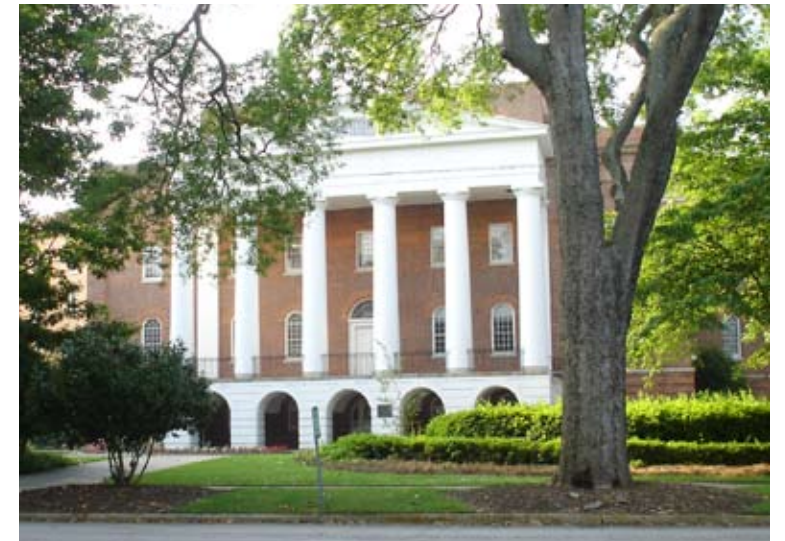
6. Cross axis of the Mills Building, North Elevation
