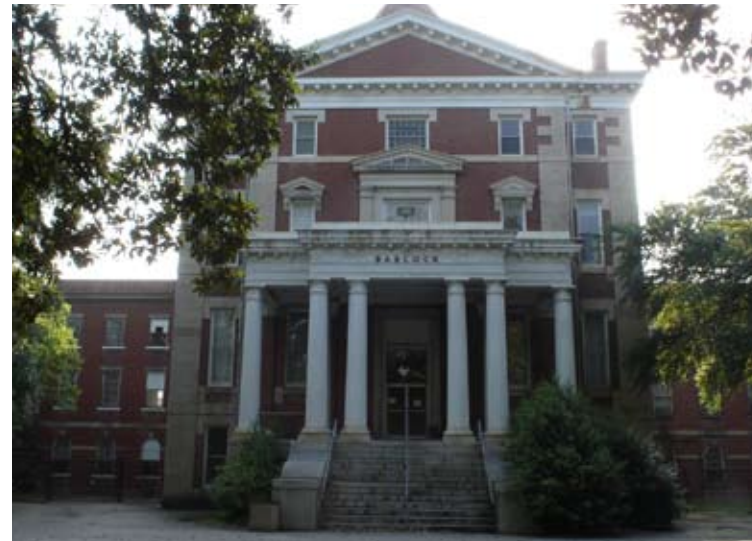
5. Babcock Building, West Elevation
