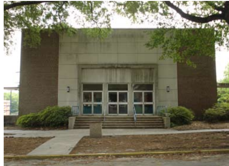
11. Benet Gymnasium and Auditorium, West Elevation
