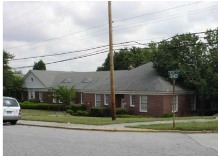
13. Wilson Building, West Elevation
