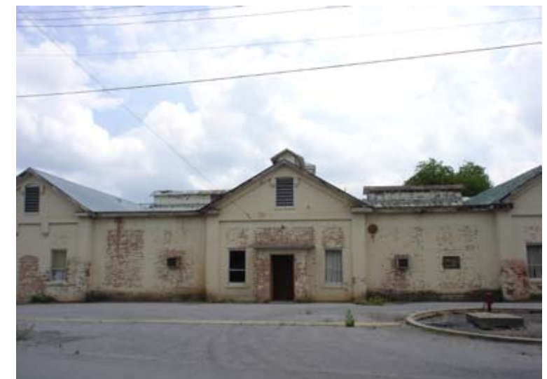
18. Storage and Laundry Building located behind the Babcock Building
