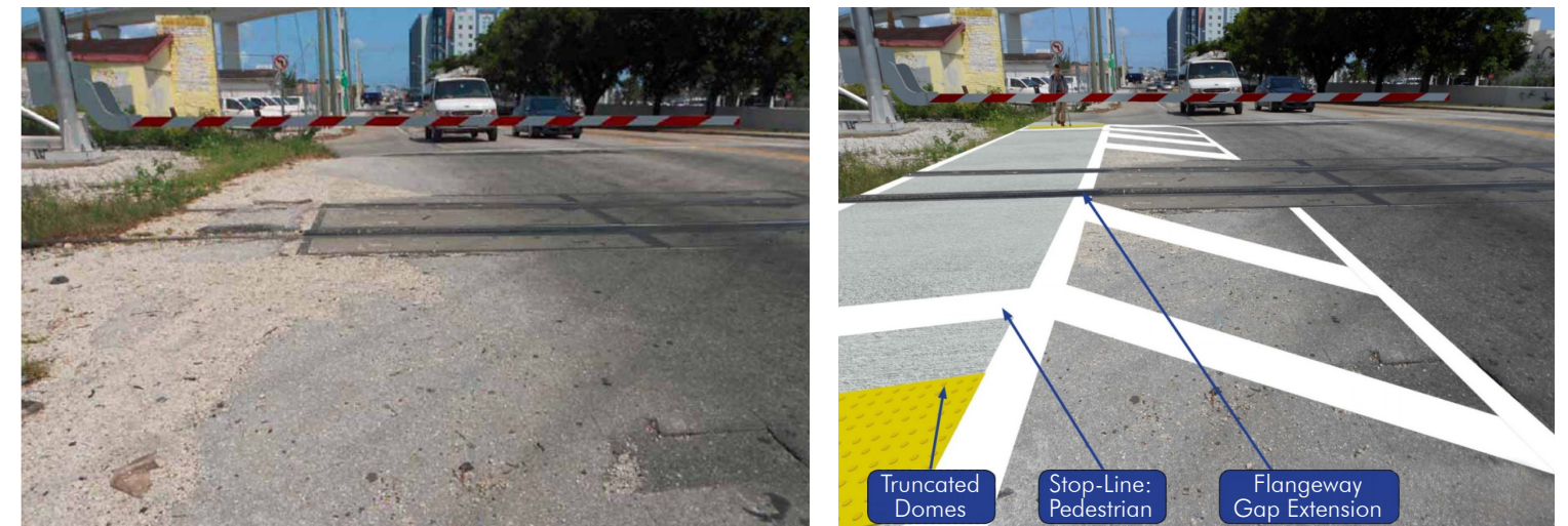
Figure 41: Before and after bike/pedestrian railroad crossing
