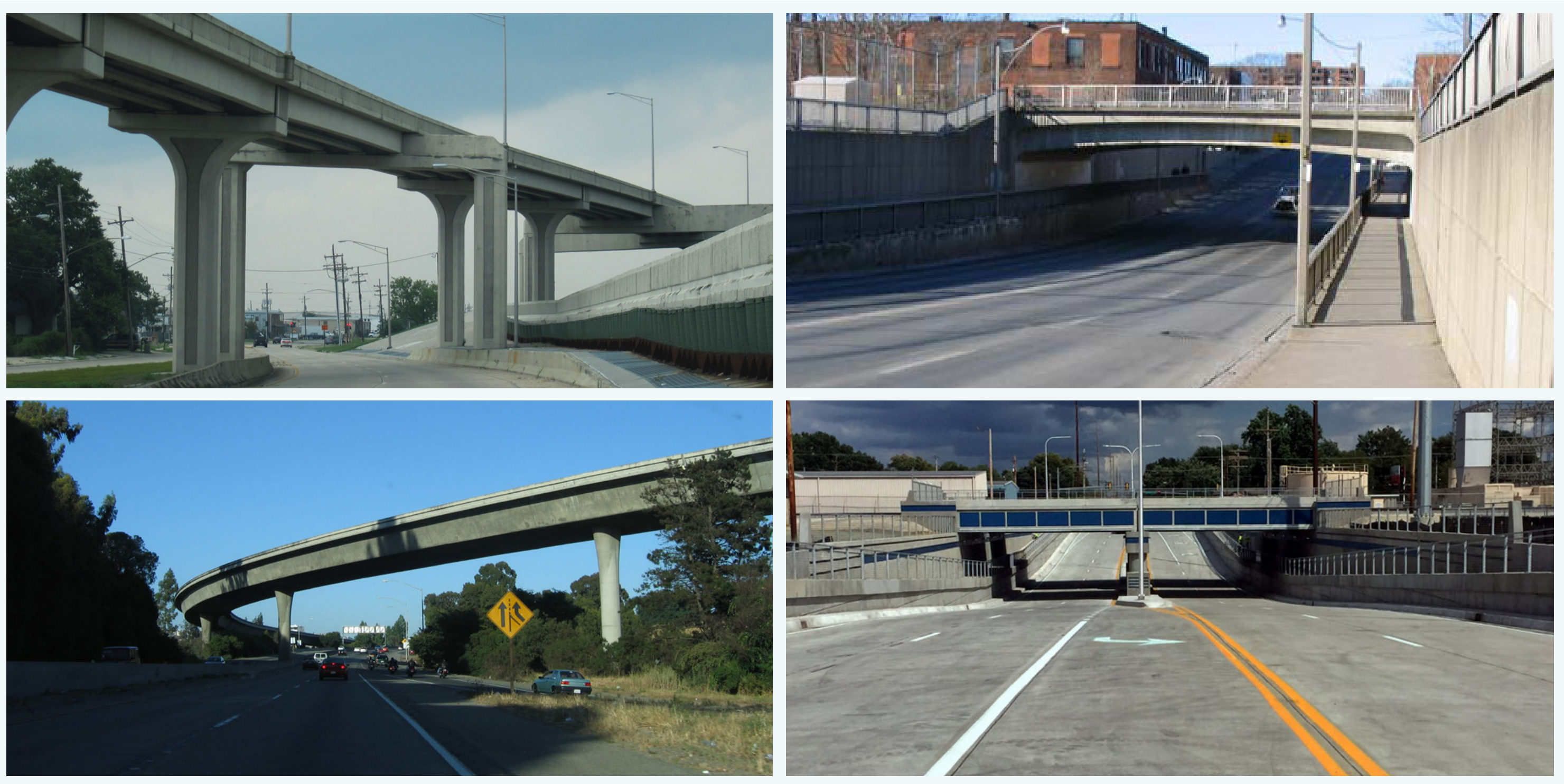
Figure 47: Examples of flyovers and underpasses
