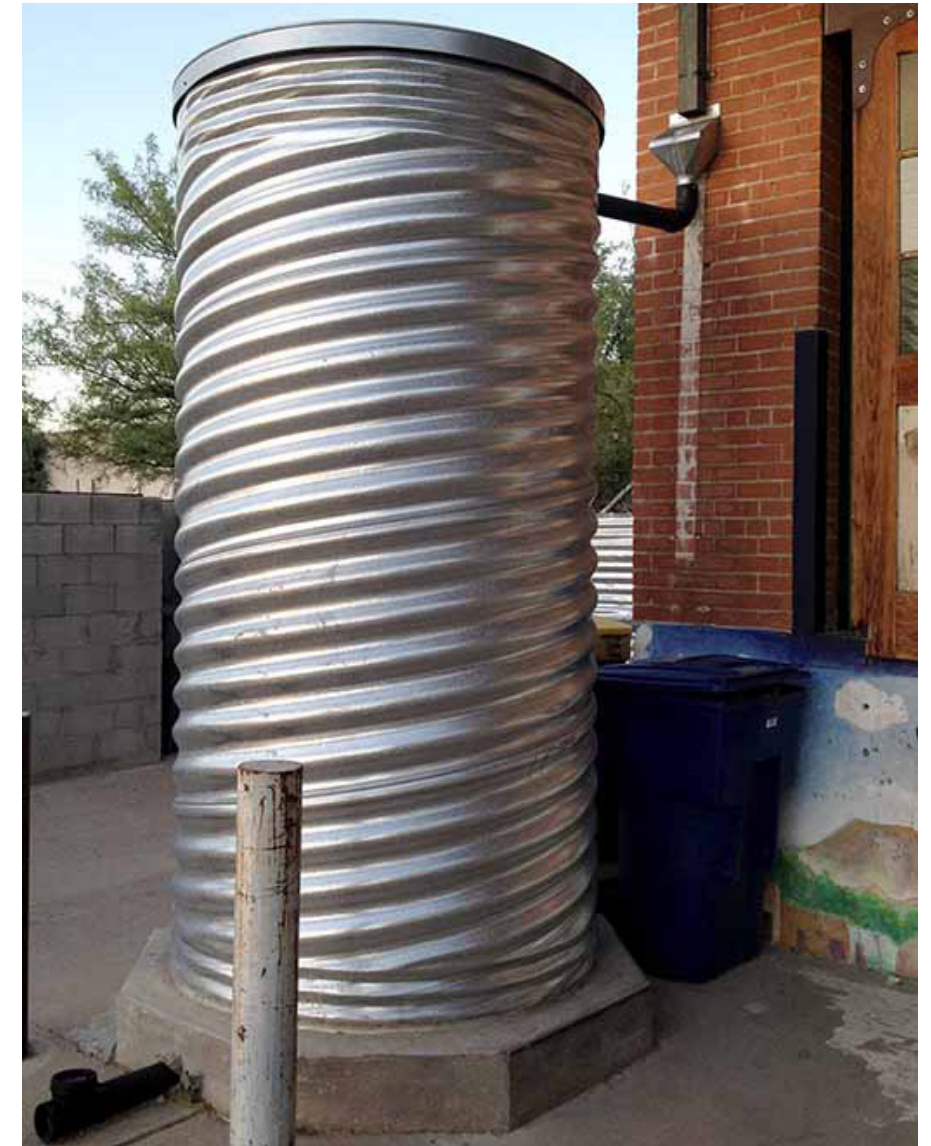
Figure 86: Cistern and/or rain barrel for rainwater harvesting
