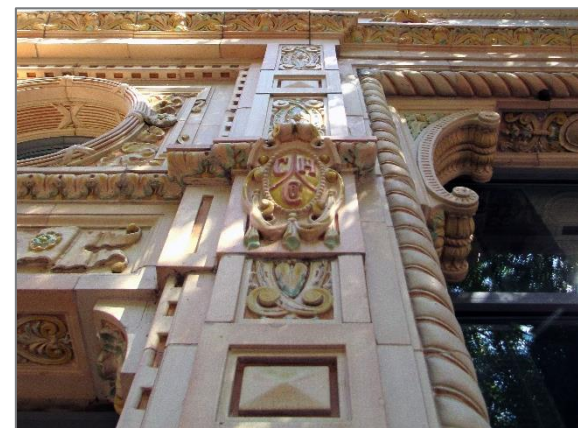
This decorative colored terracotta façade is all that remains of this historic Main Street building
