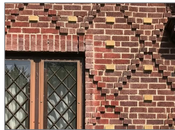
This Tudor Revival Style house in Melrose Heights uses brick diapering and colored bricks for a highly decorative effect
