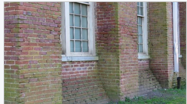
Mold, mildew, and other organic growth can be caused by a variety of problems. While cleaning will temporarily remove the problem, it does not get to the root cause. Be sure to address the source of the issue.
