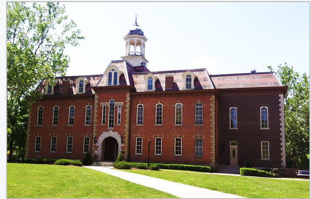
The mismatched brick discovered after building was cleaned; Photo by Richinstead.
