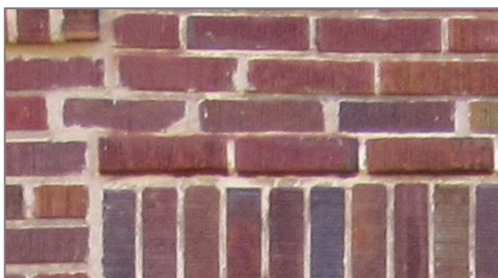
Deliberate brick details such as brick color and decorative bond patterns can be completely obscured by painting brick; Altering historic character is one of the reasons painting brick is not recommended for historic buildings.
