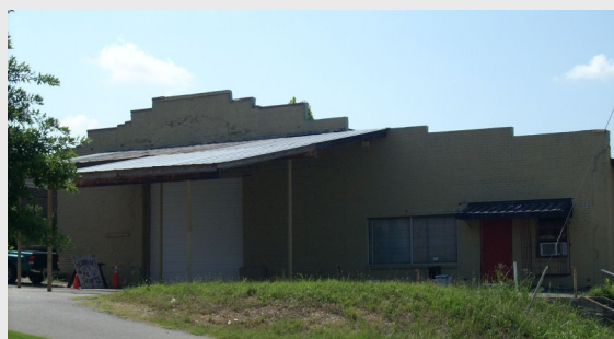
Photos of existing buildings in Innovista at the time of publication.
