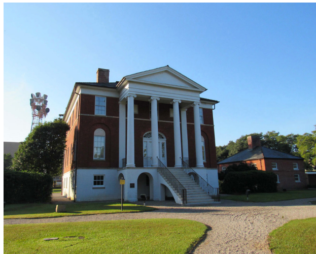
1616 Blanding Street, Robert Mills House
