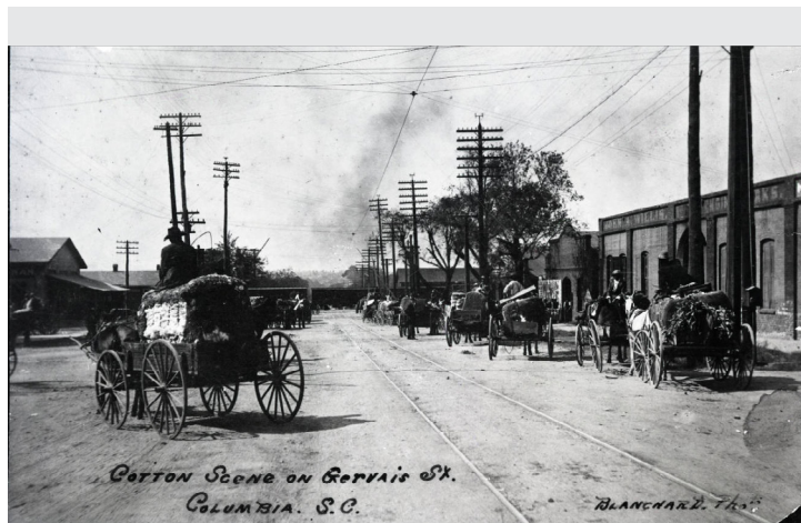
Nineteenth-century buildings in the 700 block of Gervais Street - ca. 1905 photograph. (Courtesy Richland Library)
