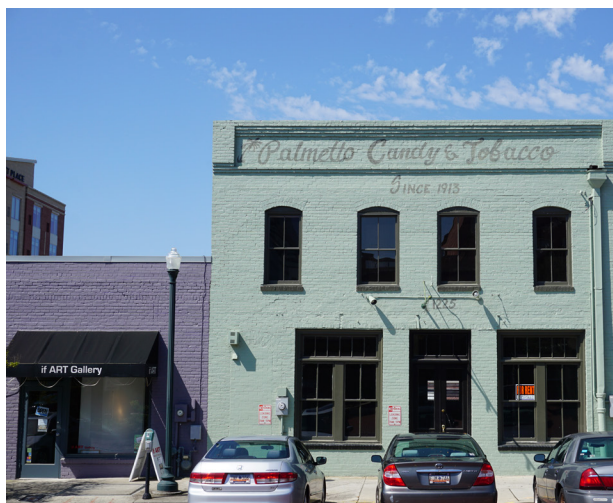
Original storefront windows and doors at 1225 Lincoln Street
