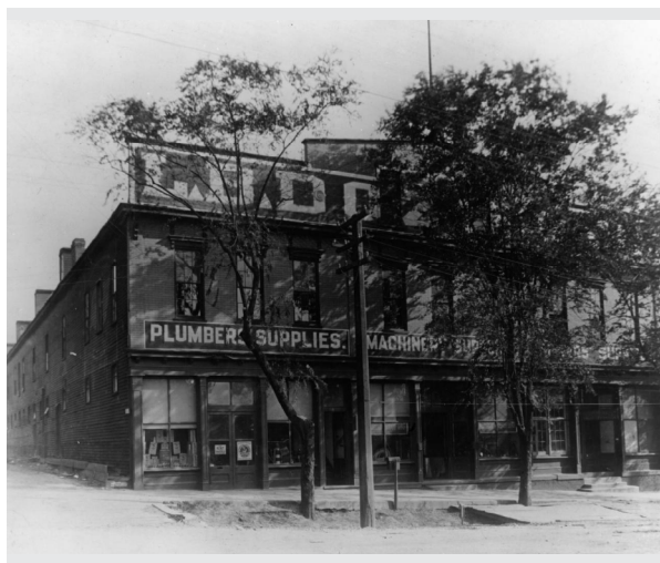
A simple, multi-bayed cast iron storefront is shown on this ca. 1906 image of 810-816 Gervais Street, which was perhaps the earliest multi-story retail building in the Vista. (Courtesy Richland Library)
