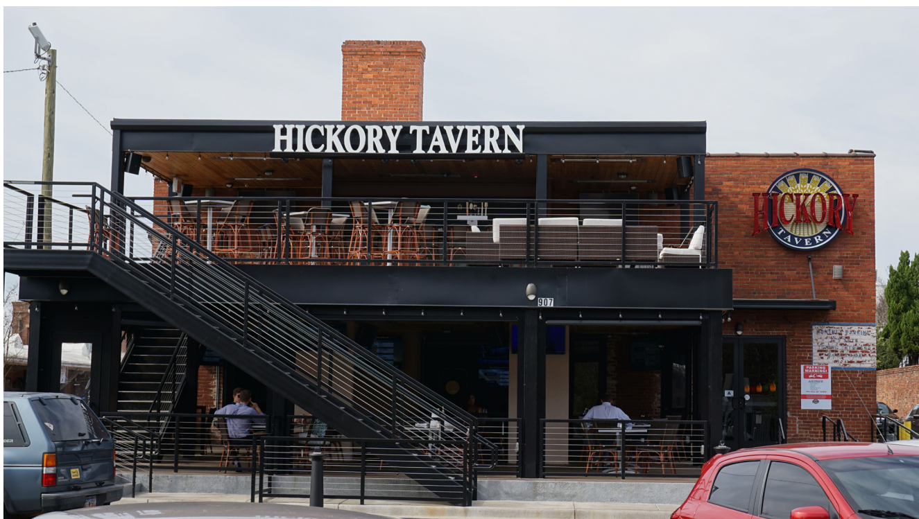
Porch addition to the rear of 912 Gervais Street
