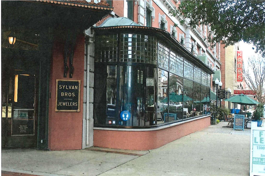
Photo 4 – Prism glass transom and curved display windows, looking east
