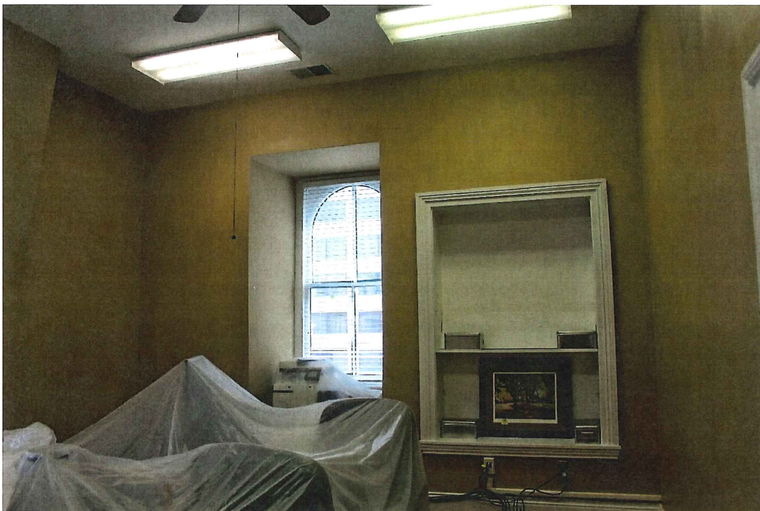
Photo 49 – Third floor office, looking south
