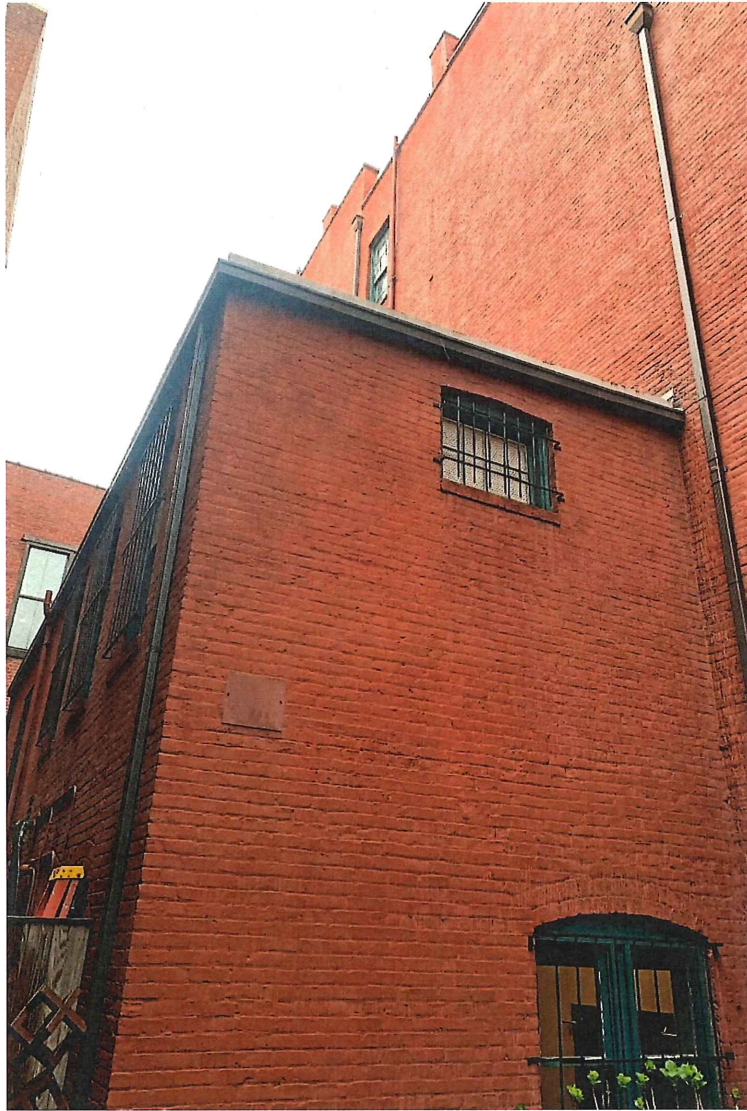
Photo 11 – North elevation, looking east
