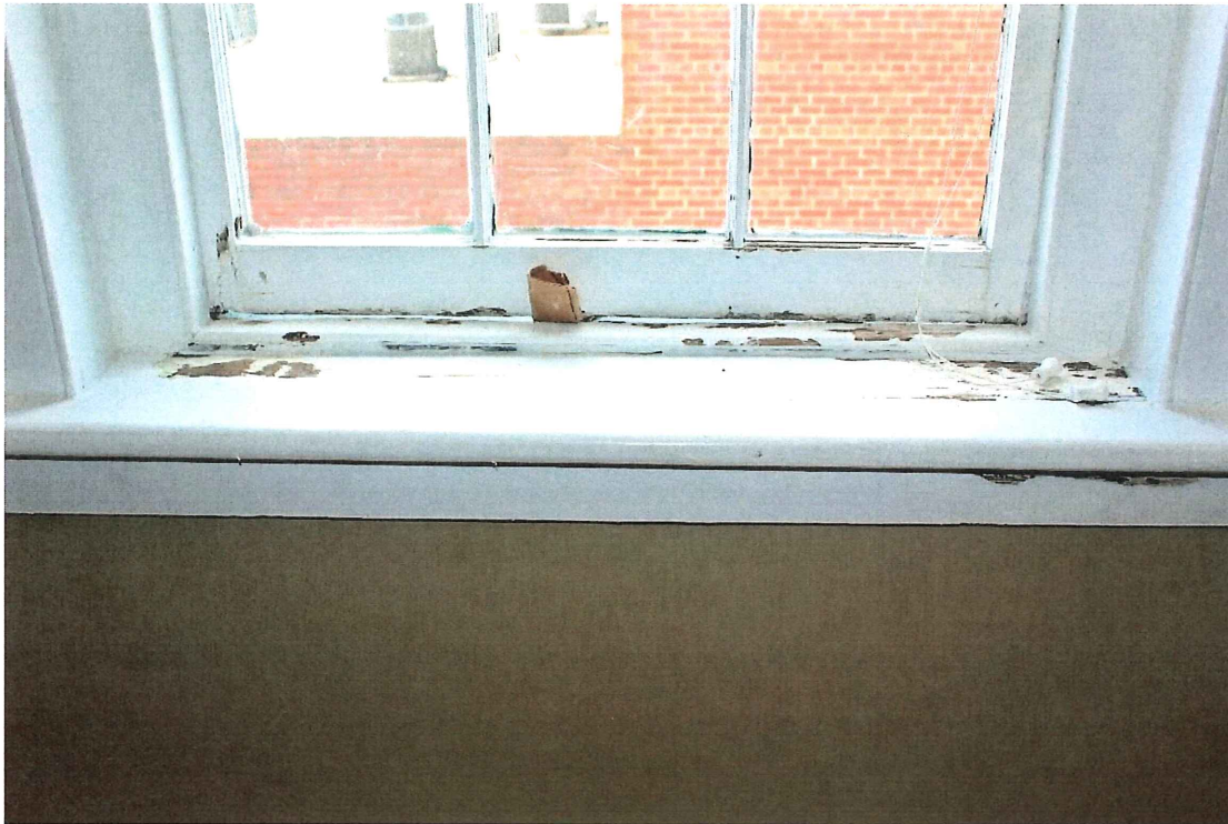
Photo 48 – Third floor window detail, looking north
