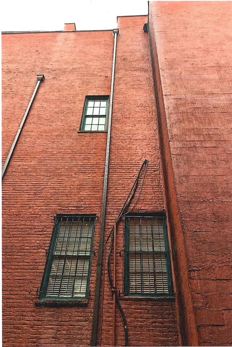
Photo 9 – North elevation brick and windows
