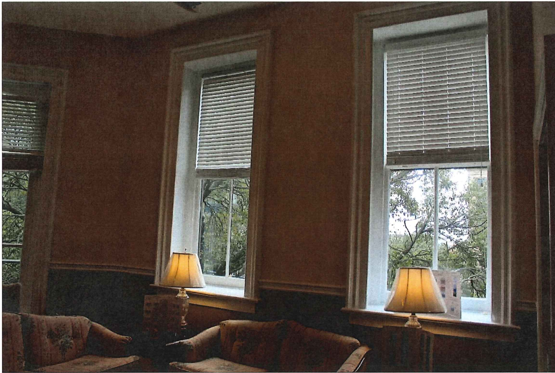
Photo 30 – Second floor office, looking west
