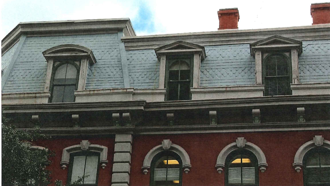
Photo 14 – Dormers on western end of south elevation
