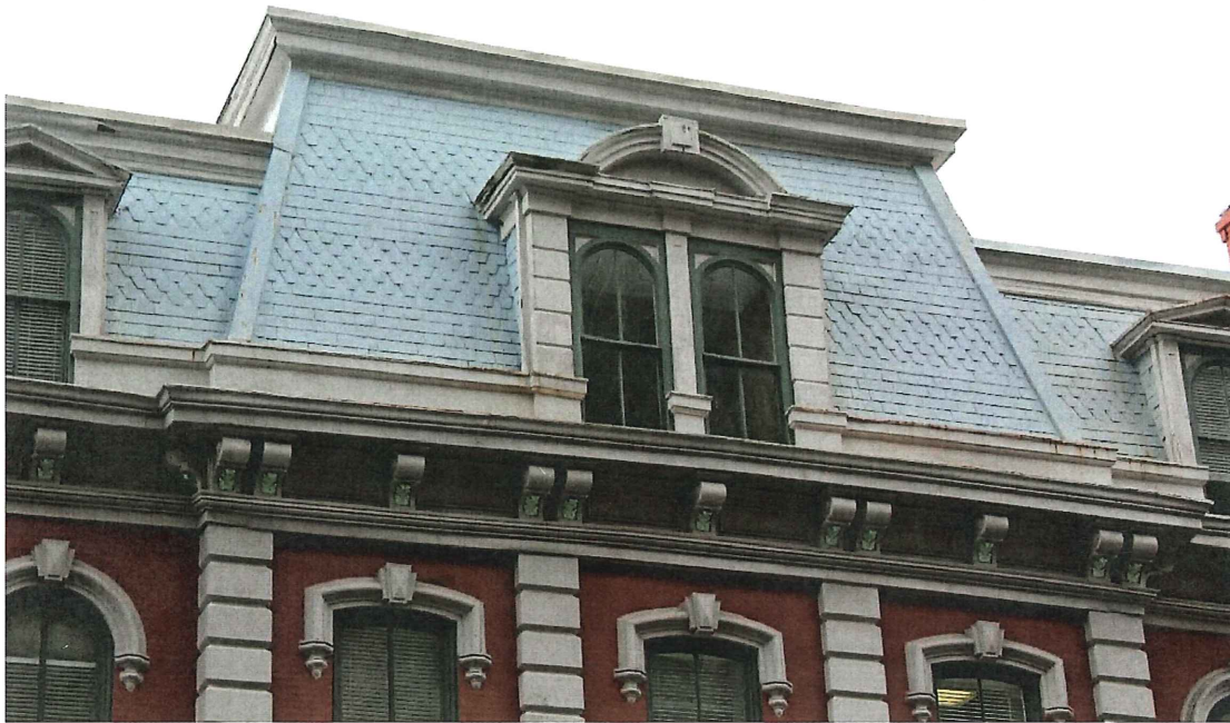
Photo 13 – Center dormer on south elevation
