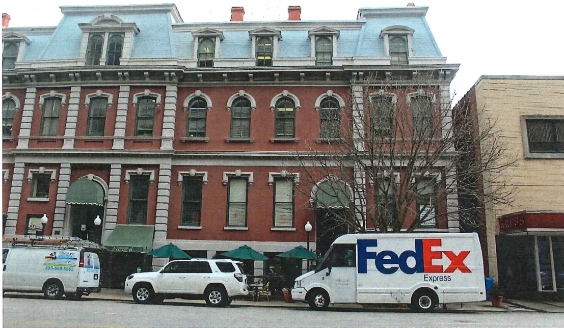
Photo 5 – East end of south elevation, looking north
