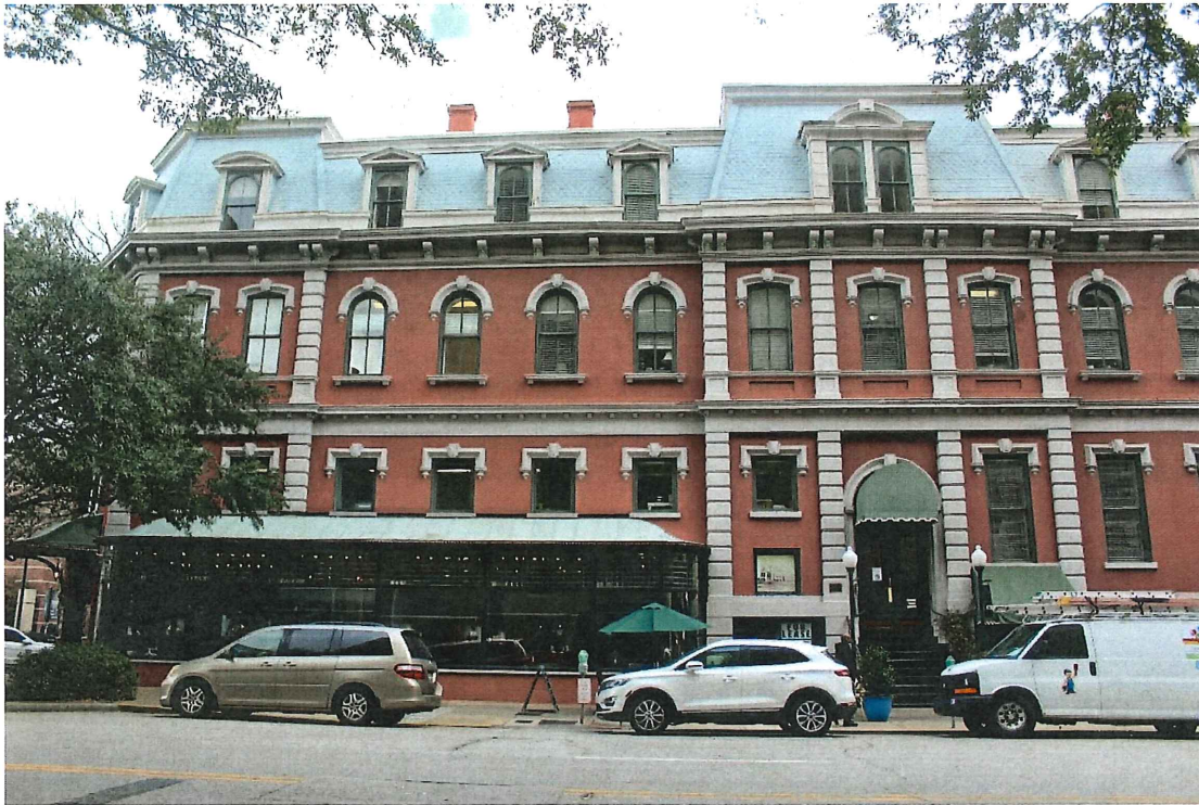
Photo 3 – West end of south elevation, looking north
