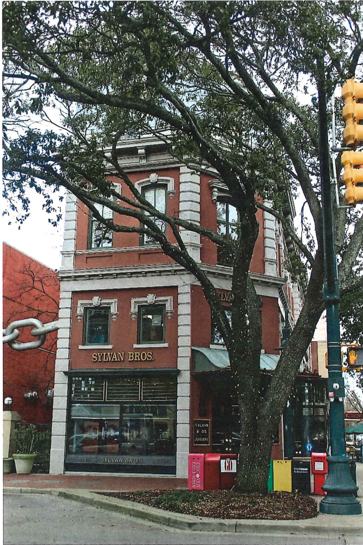
Photo 7 – West elevation and corner entrance, looking east
