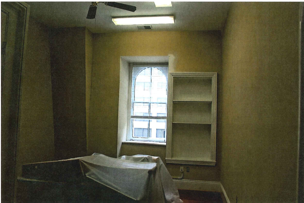
Photo 47 – Third floor office, looking south
