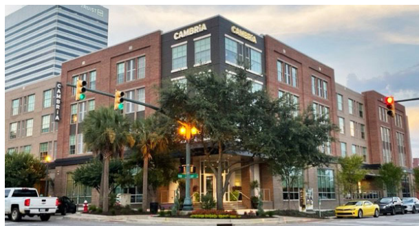
1000 Lady Street: Approved in 2020, the Cambria Suites Hotel on Lady Street completed construction in 2022. The wide sidewalk at the corner invites guests with a canopy over the recessed corner entrance, shade from nearby street trees, and welcoming lighting and potted plants around the front door. The massing of the building along both streets is broken up into smaller structural bays to add interest to the street and respond to the scale of nearby historic buildings.
