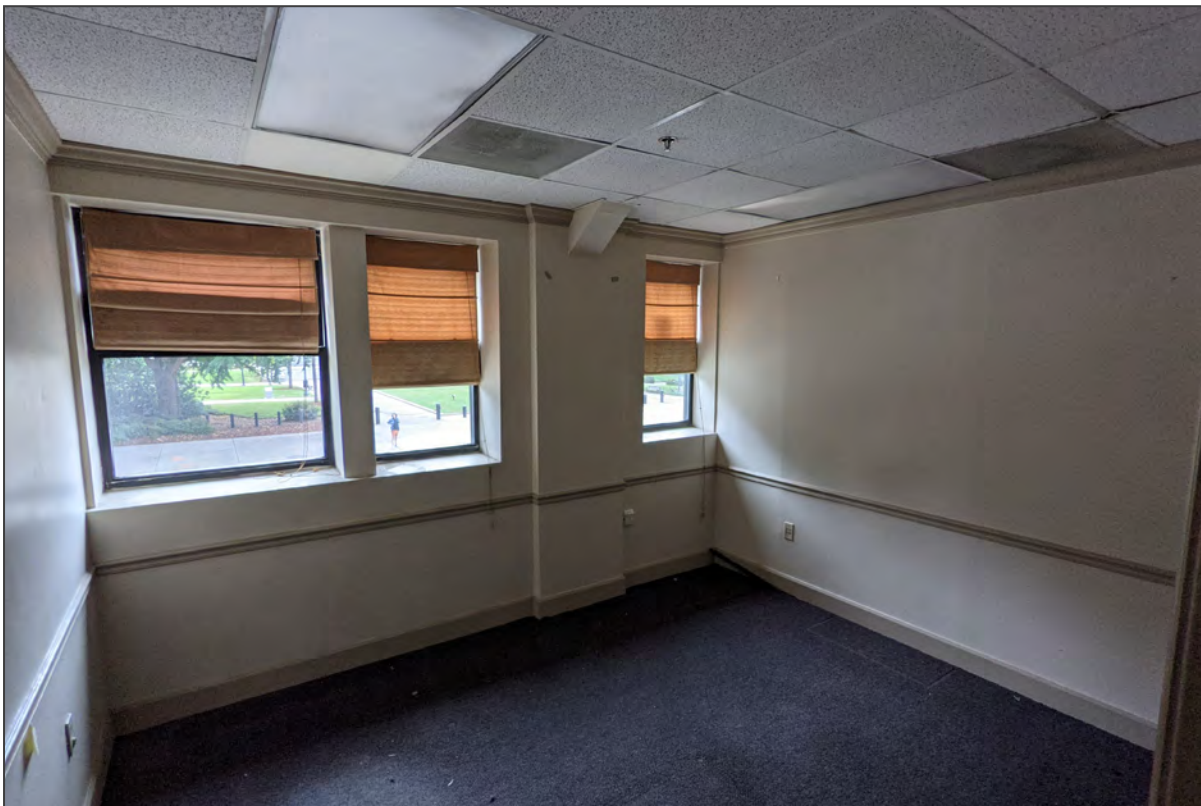
47. Mezzanine/second floor, west office, view south
