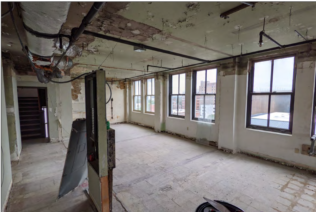
63. Sixth floor, view north towards staircase
