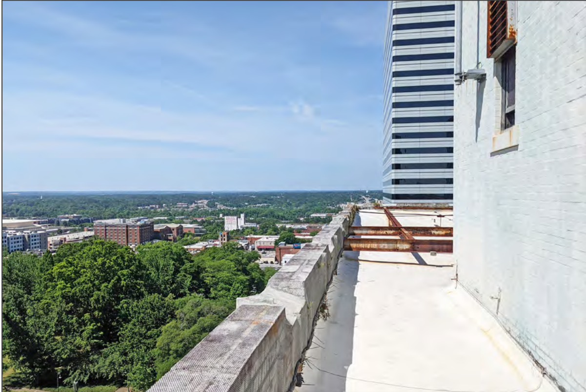
109. Roof, view southwest
