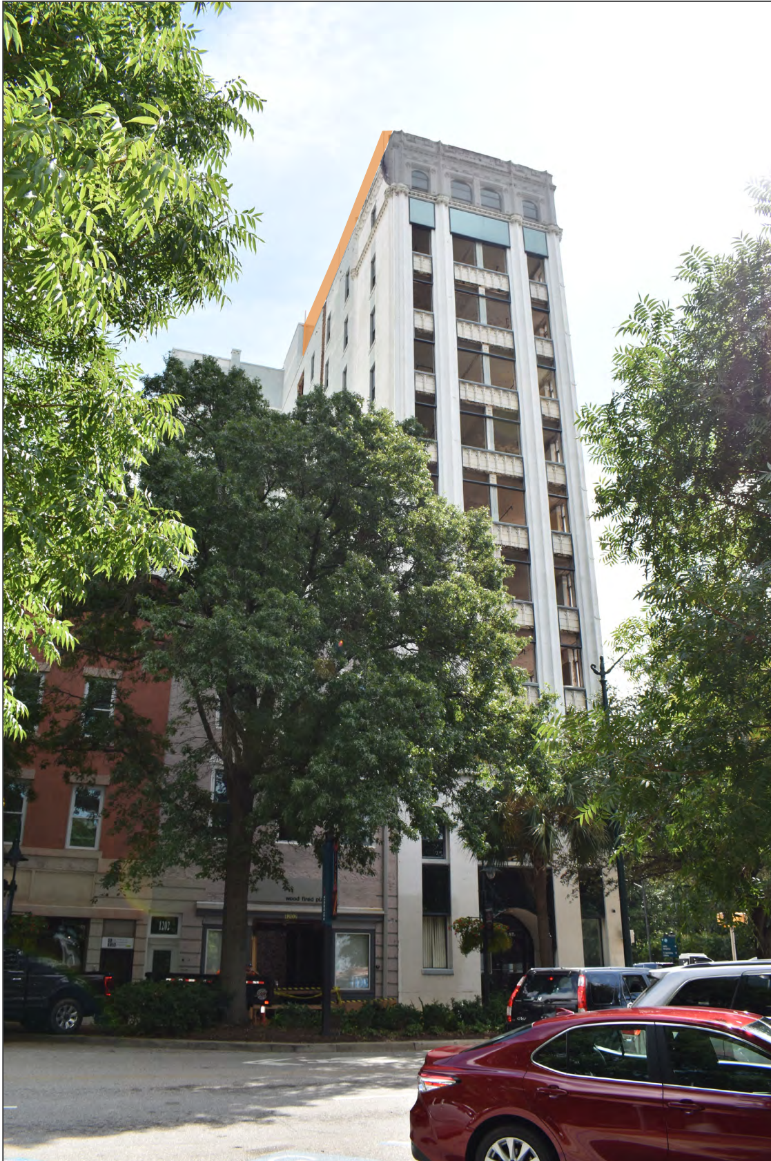
127. Rooftop Bar Mock-up (highlighted in orange), view west
