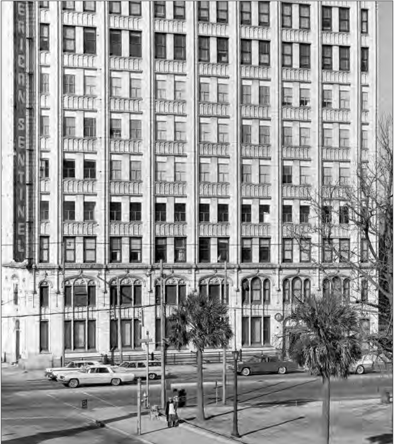
Historic Image H. 1962 photo of Gervais Street elevation. Photo shows a mix of original and replacement windows. Courtesy of the Richland County library.
