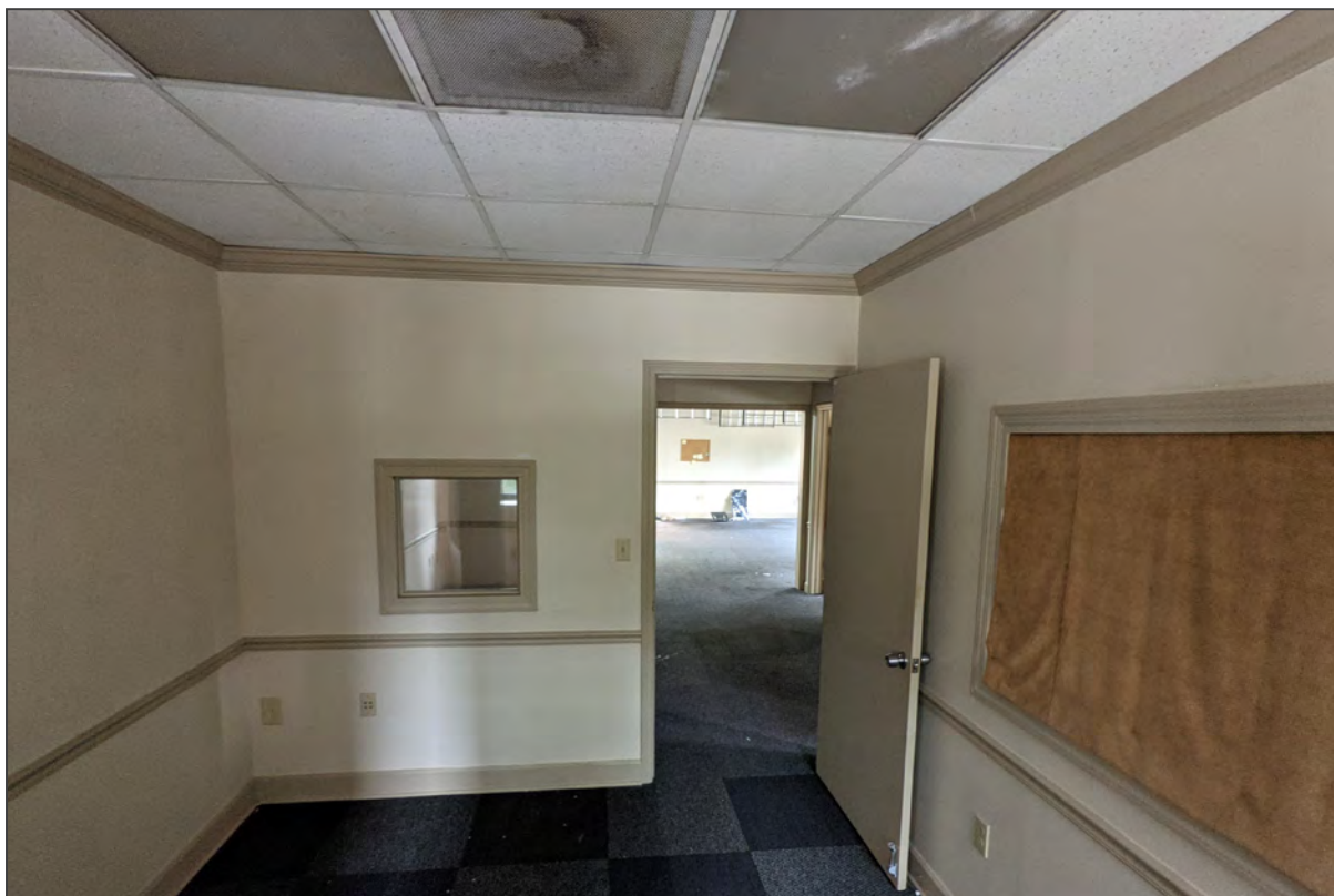
53. Mezzanine/second floor, northwest office, view east
