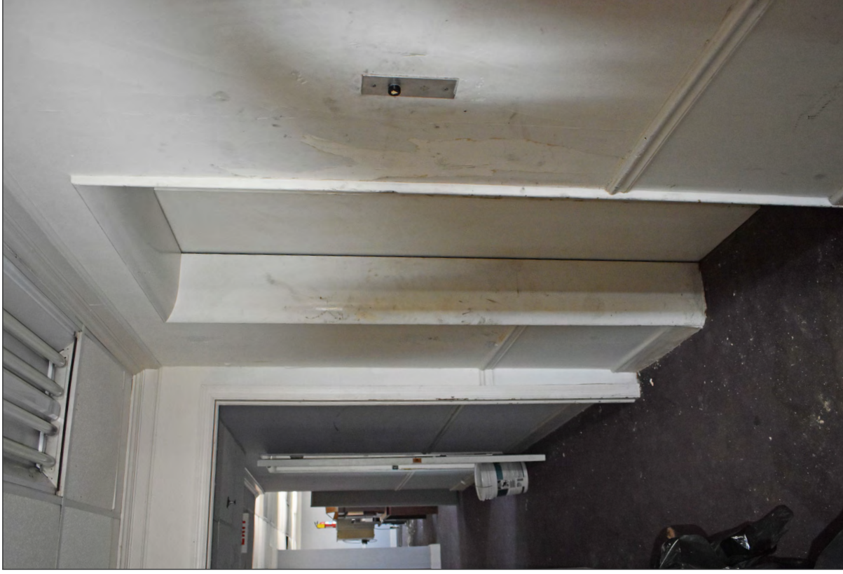
97. Eleventh floor, elevator lobby, view northwest
