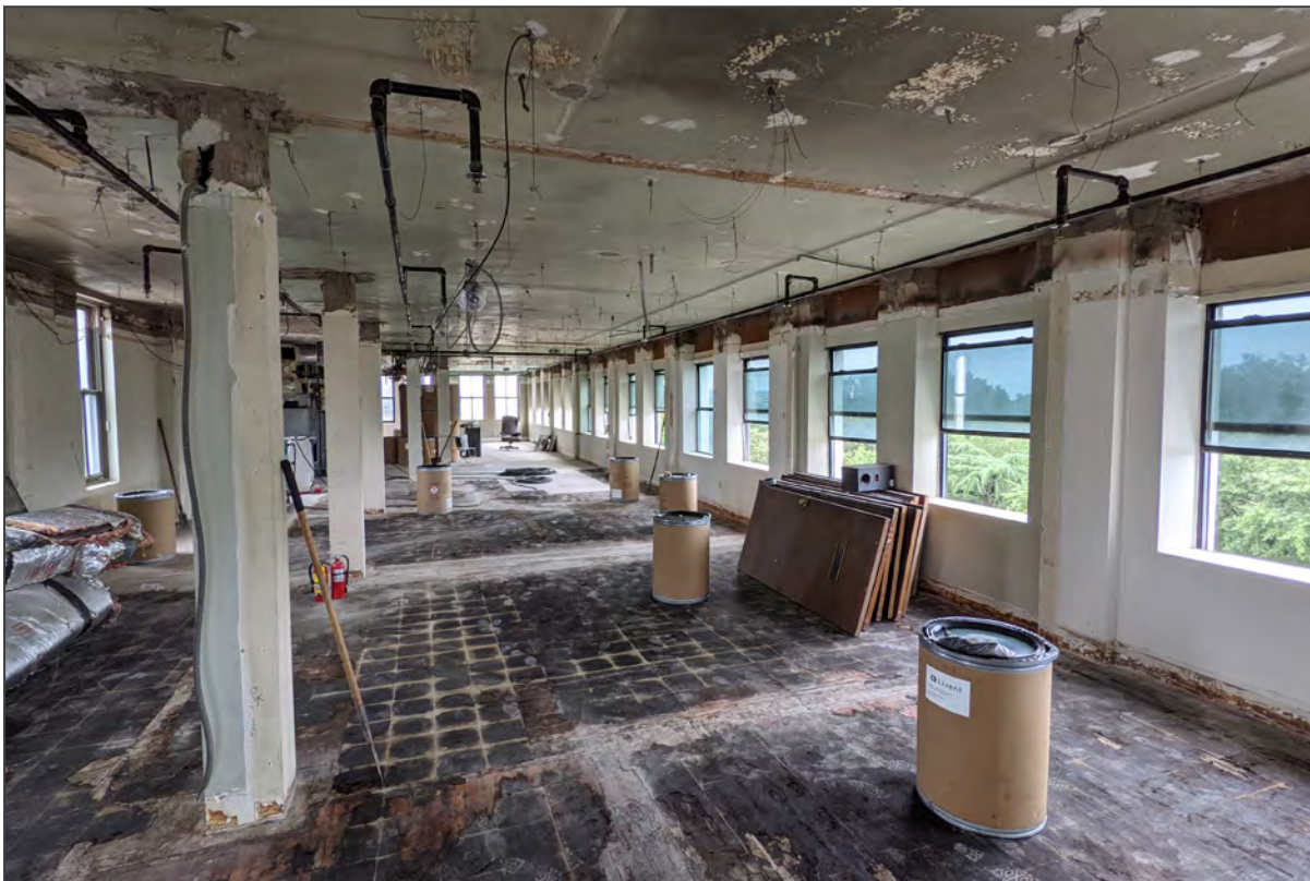
61. Sixth floor, view east
