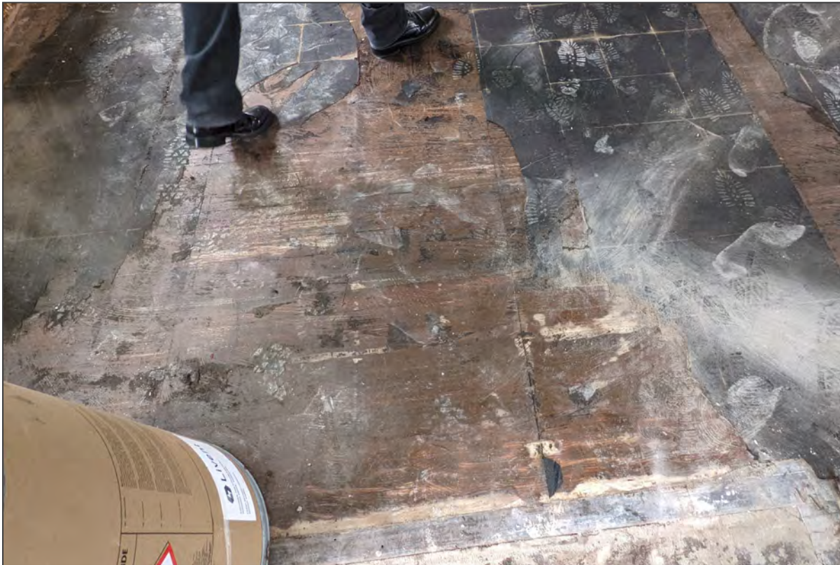
64. Sixth floor, historic wood flooring example
