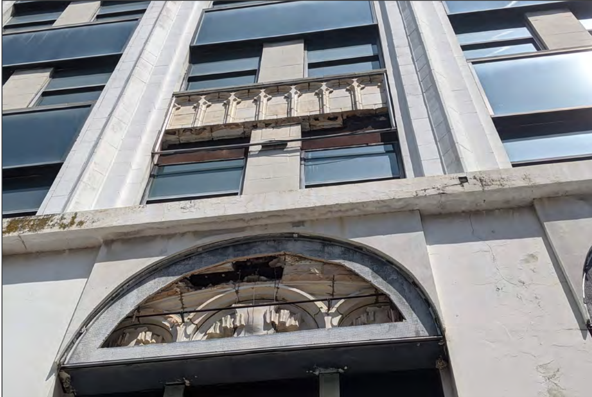
10. South elevation, historic terra cotta details
