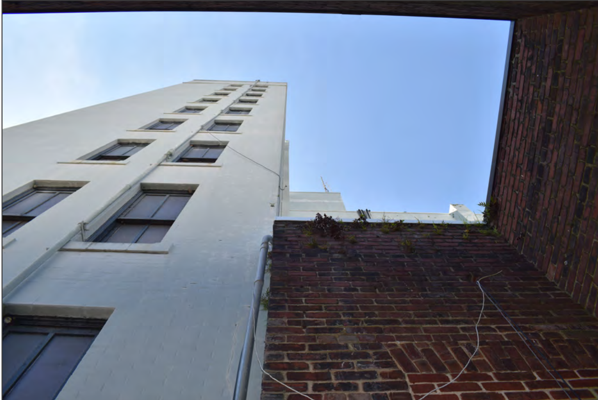
18. North elevation, view southeast
