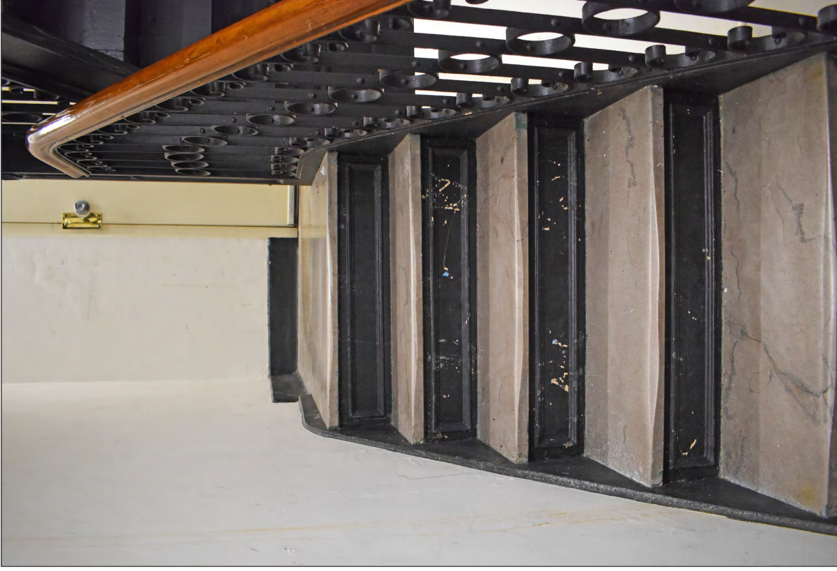
83. Staircase, view north
