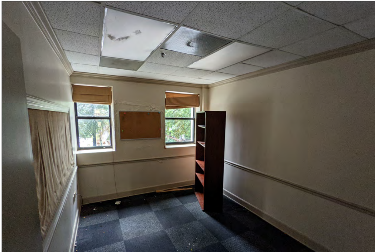
52. Mezzanine/second floor, northwest office, view northwest
