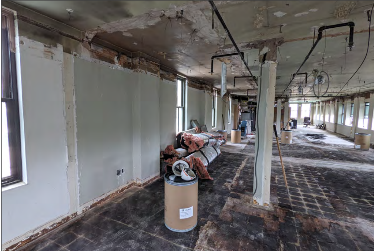
62. Sixth floor, view northeast
