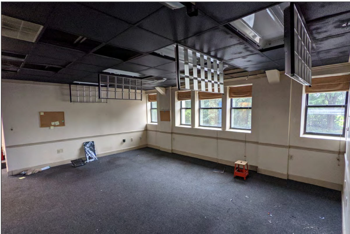
45. Mezzanine/second floor, open office, view southeast
