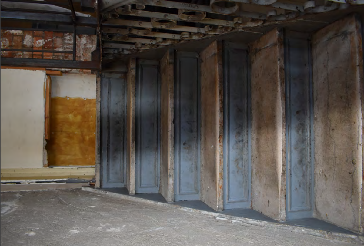
34. First floor, staircase to basement, view north
