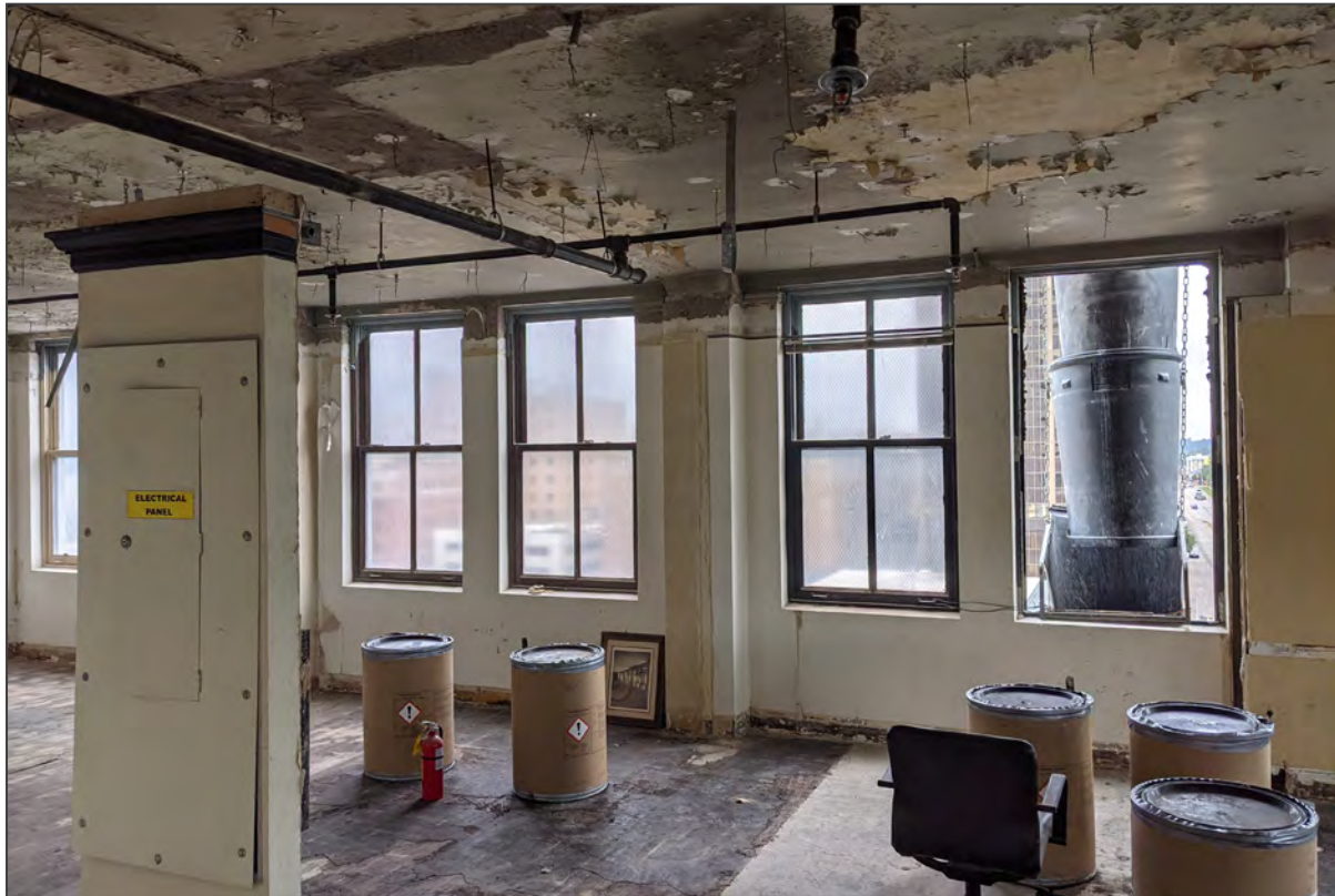
66. Seventh floor, view northeast
