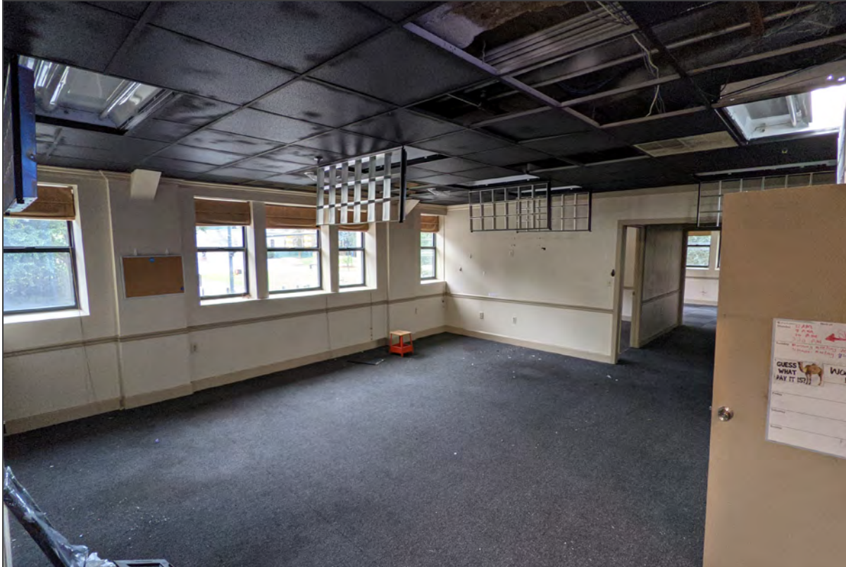
44. Mezzanine/second floor, open office, view southwest
