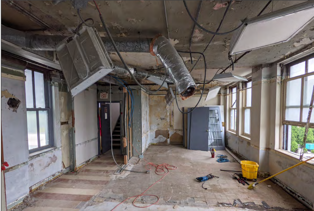
60. Fourth floor, historic hallway terrazzo at left, view north towards staircase
