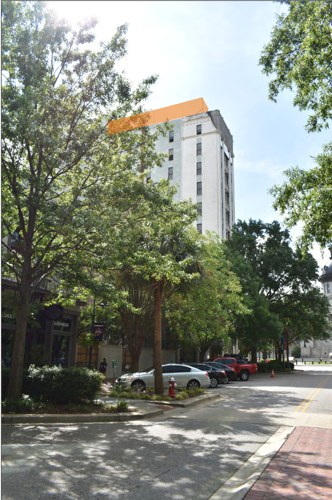
128. Rooftop Bar Mock-up (highlighted in orange), view southeast
