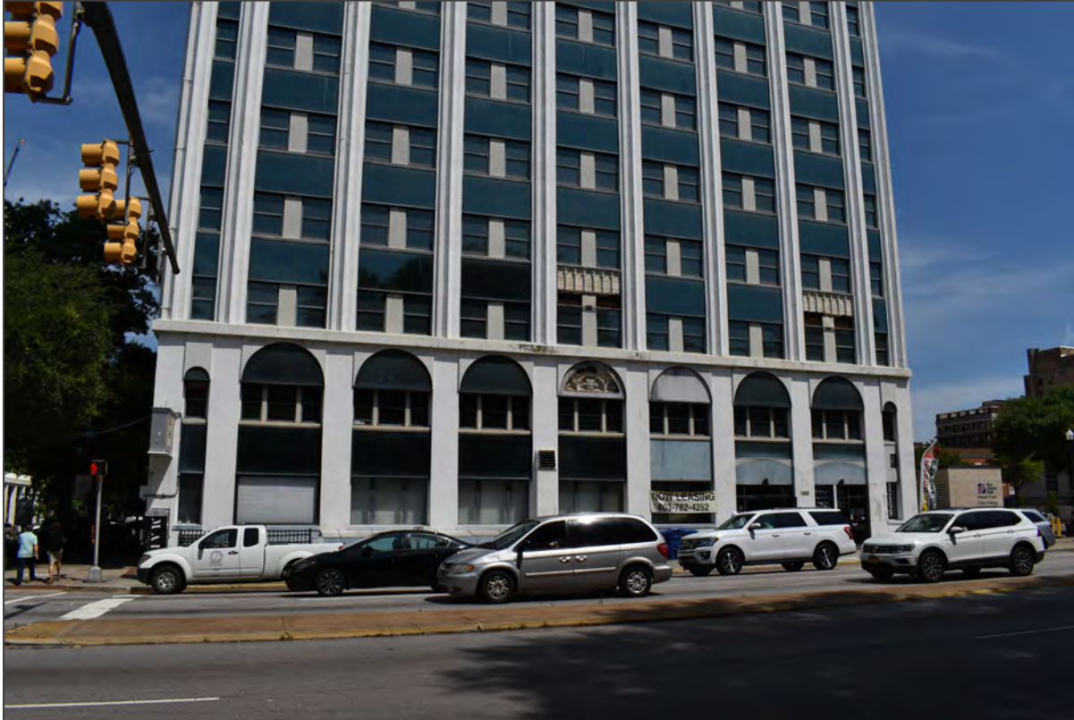
8. South elevation, bottom floors, view north
