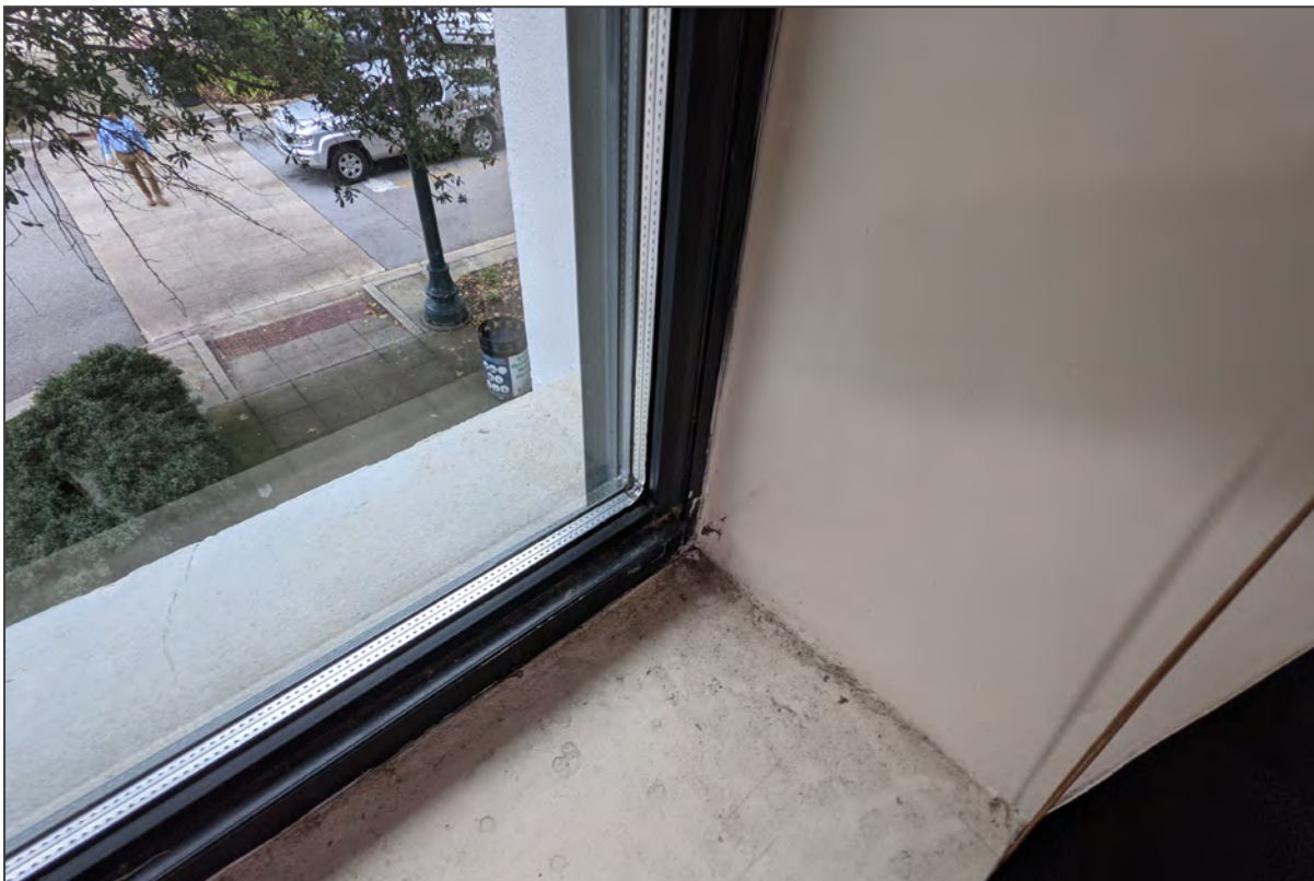
51. Mezzanine/second floor, southwest office, window sill
