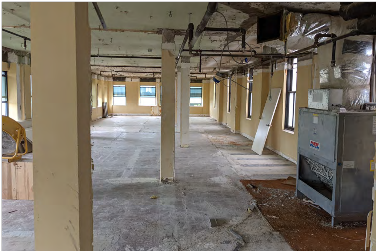
67. Eighth floor, view west
