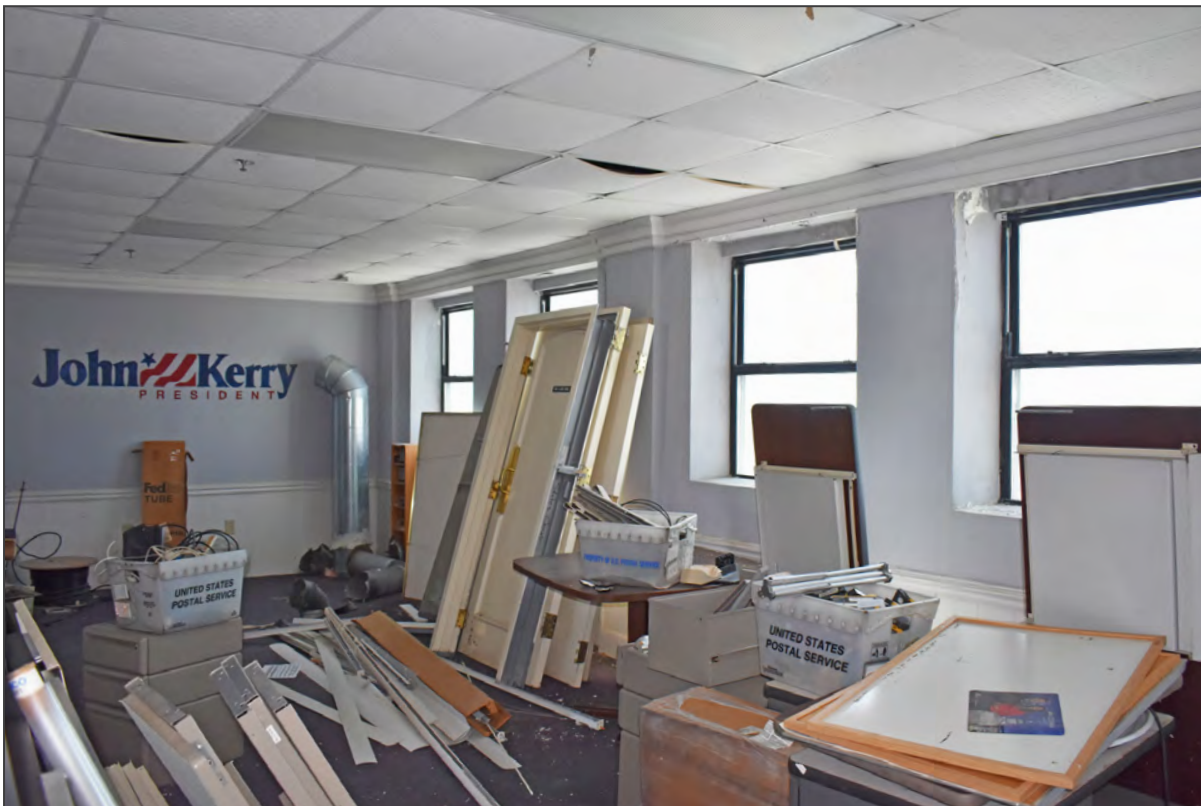
102. Eleventh floor, south office, view southeast
