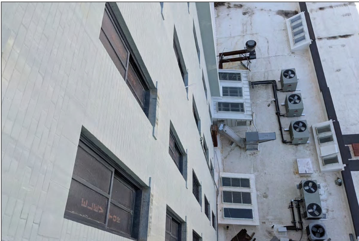
19. North elevation, looking down on roof of 1202 Main, view southwest
