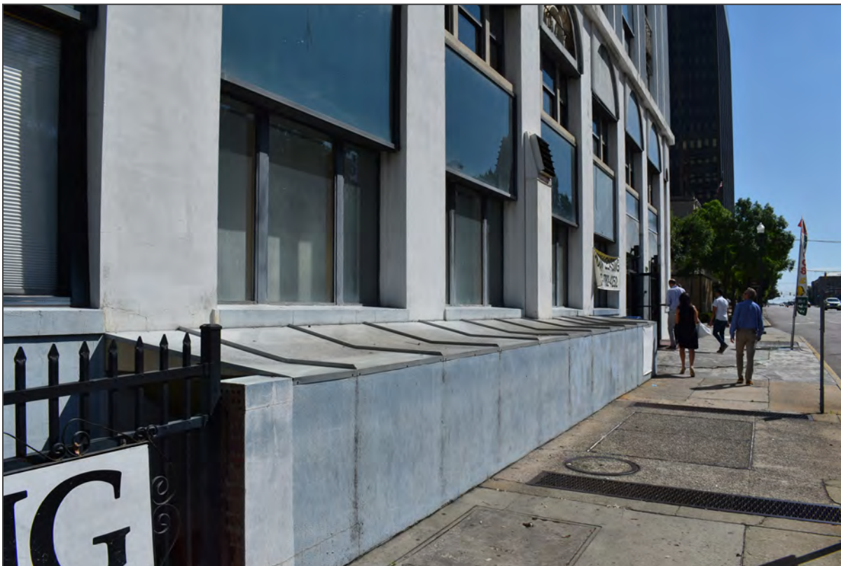
9. South elevation, first floor, view northeast
