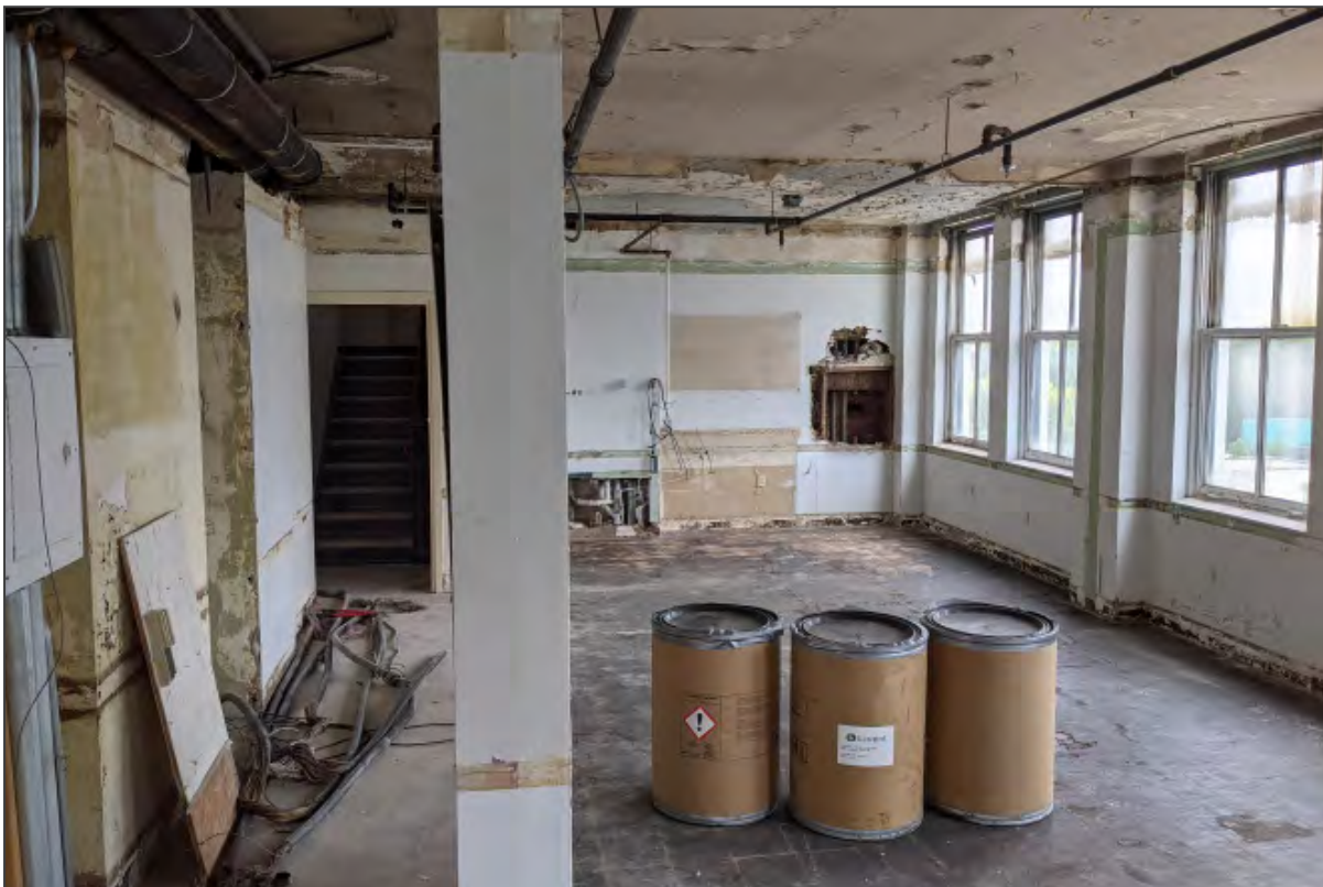
55. Third floor, view north towards staircase
