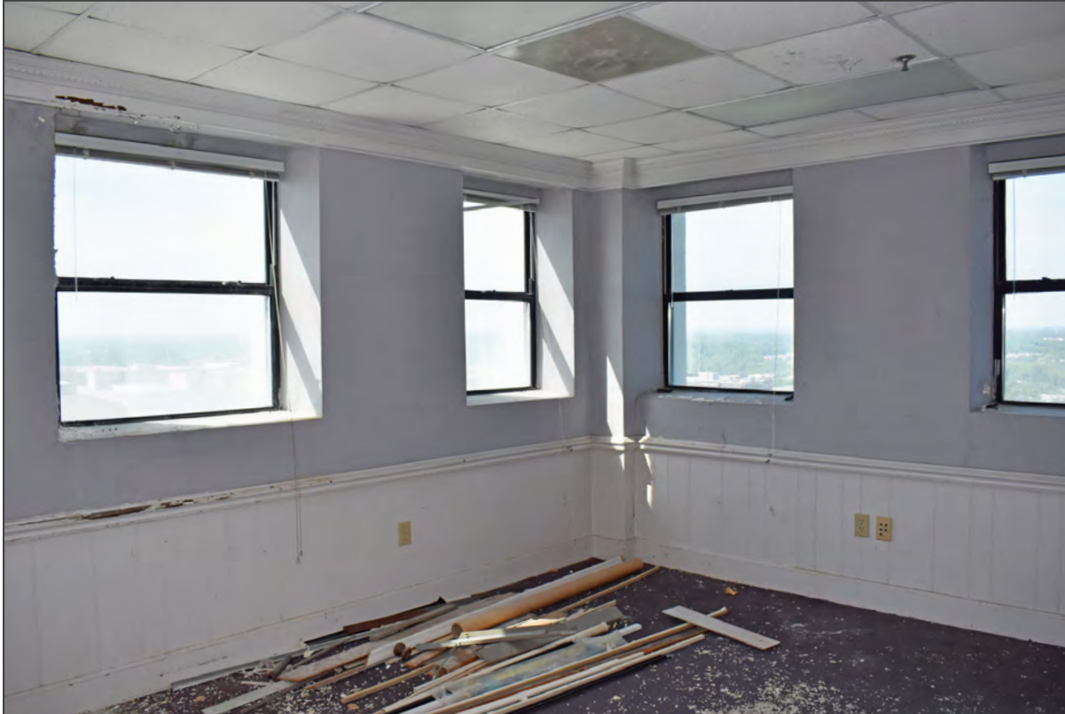
103. Eleventh floor, west office, view southwest
