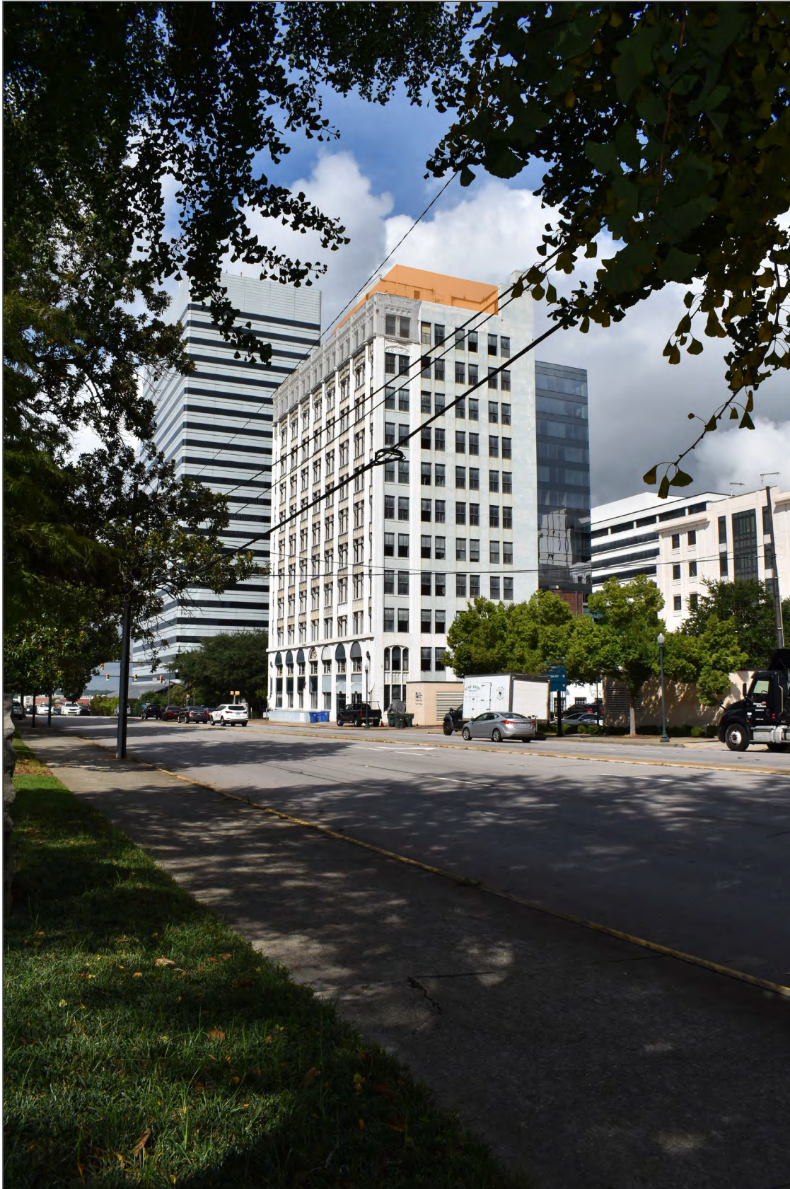
125. Rooftop Bar Mock-up (highlighted in orange), view east
