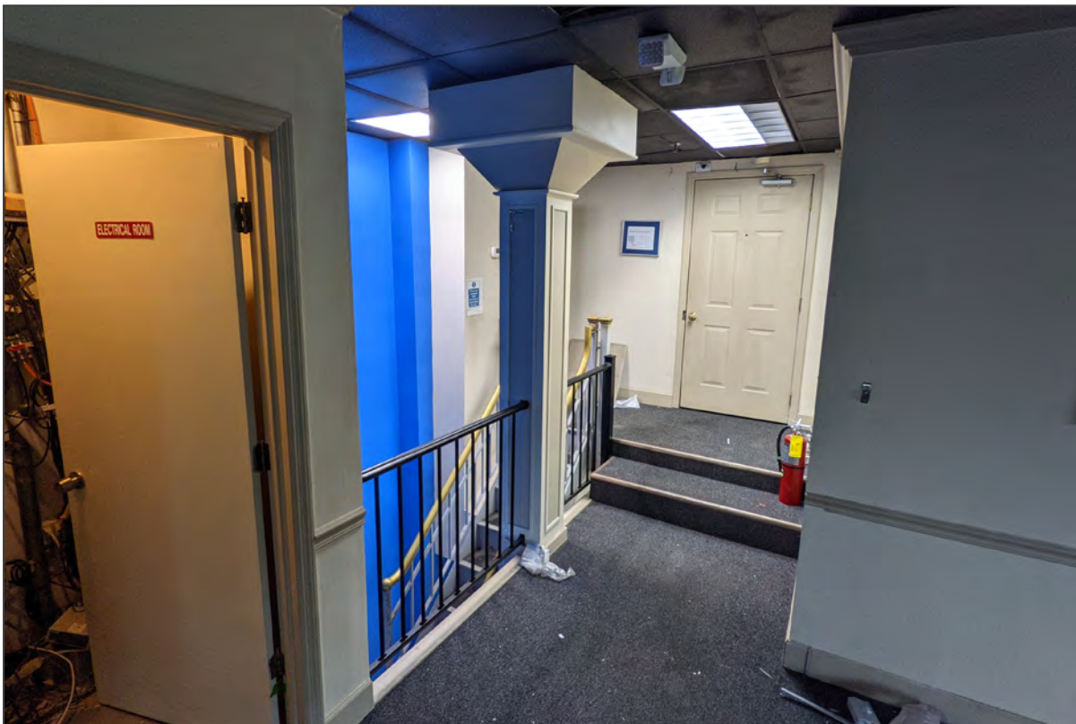
43. Mezzanine/second floor, staircase hallway, view northeast
