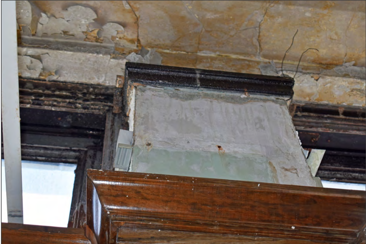
81. Ninth floor, northeast office, older molding visible above current drop-ceiling framing
