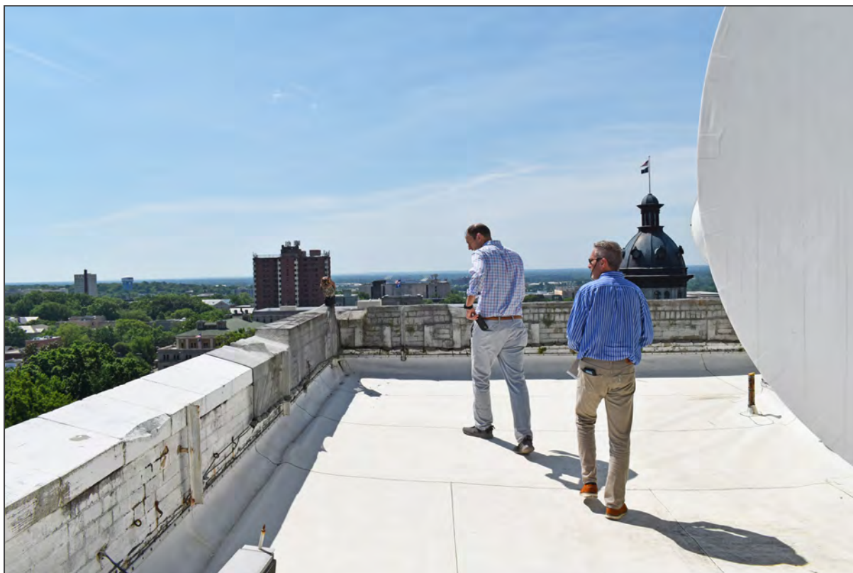
108. Roof, view southeast
