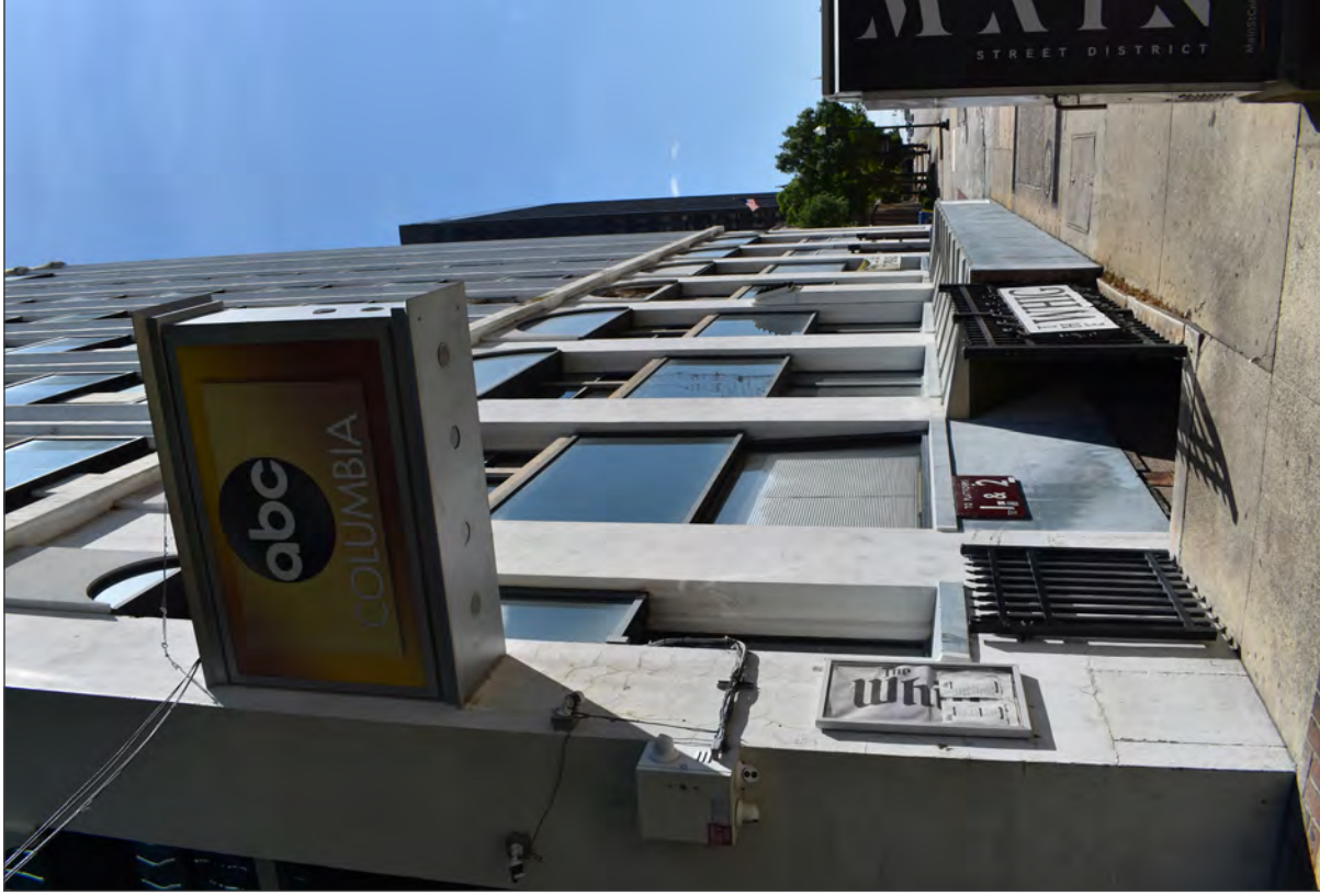
6. South elevation, view northeast
