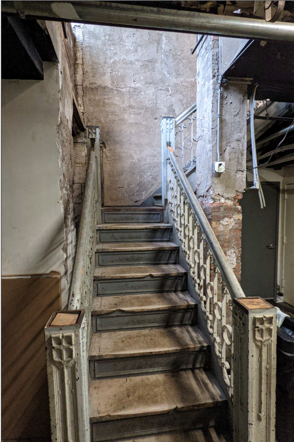
21. Basement, staircase to first floor
