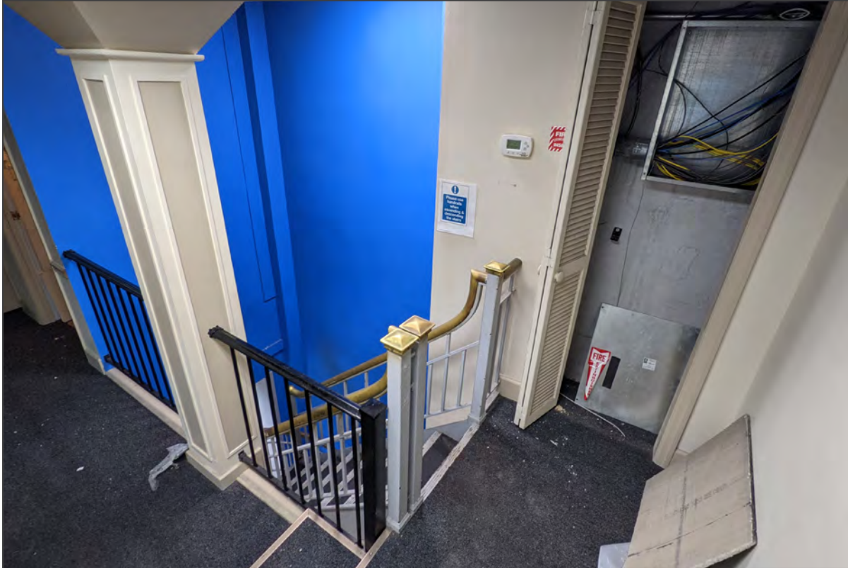
42. Mezzanine/second floor, staircase to first floor, view northwest
