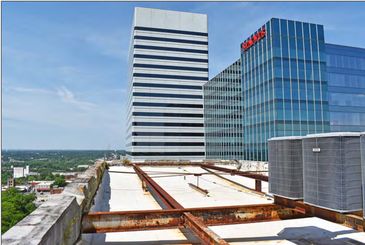
111. Roof, view west
