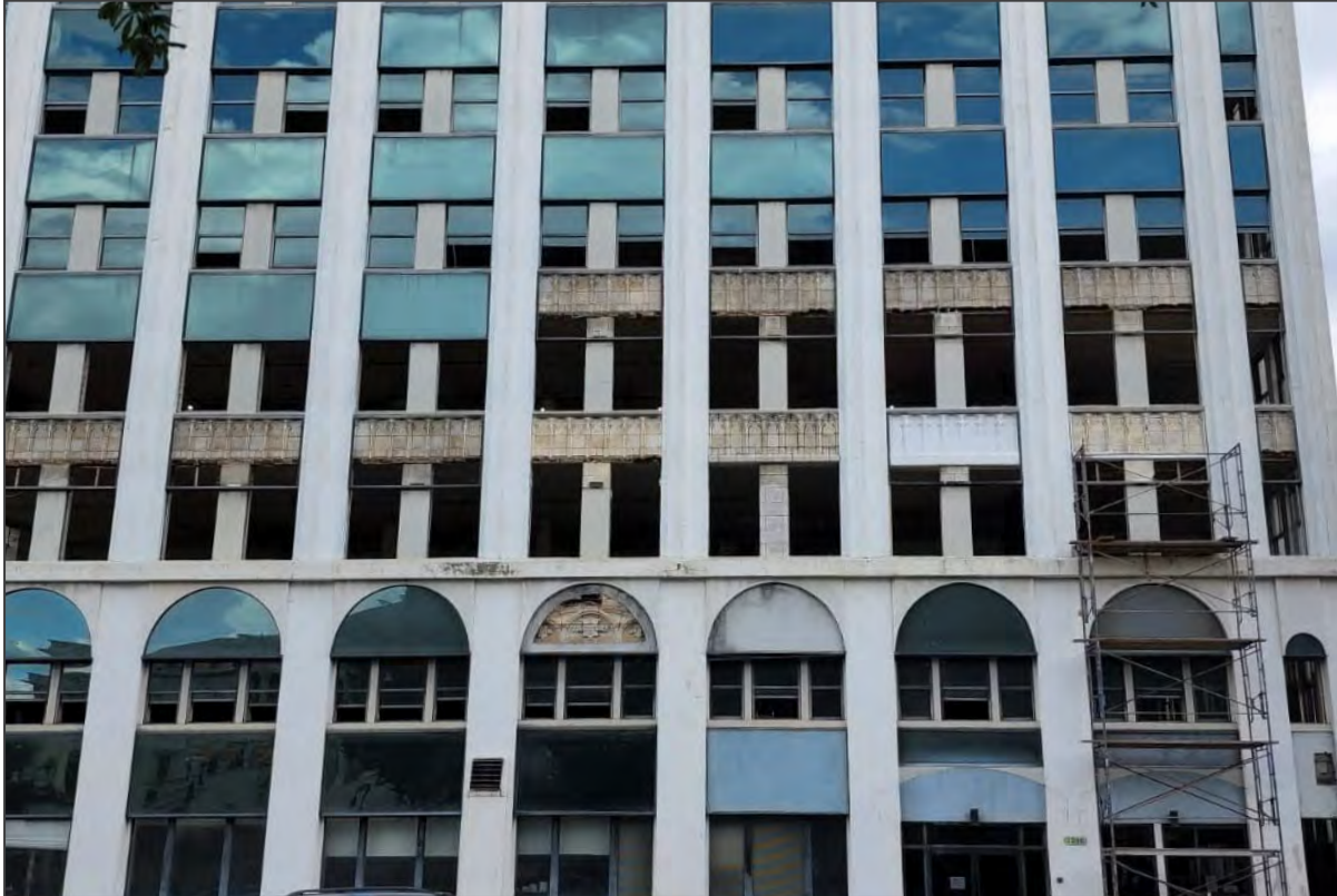
118. Uncovered terra cotta tiles, with test replacement panel second from right.
