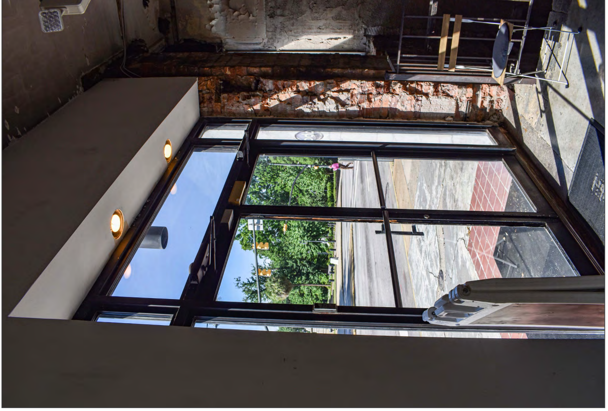
36. First floor, Gervais Street main entrance, view southwest
