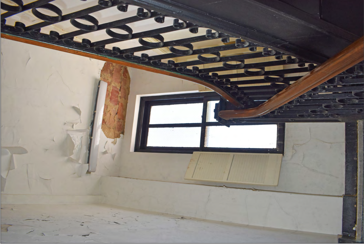
84. Staircase, view northeast
