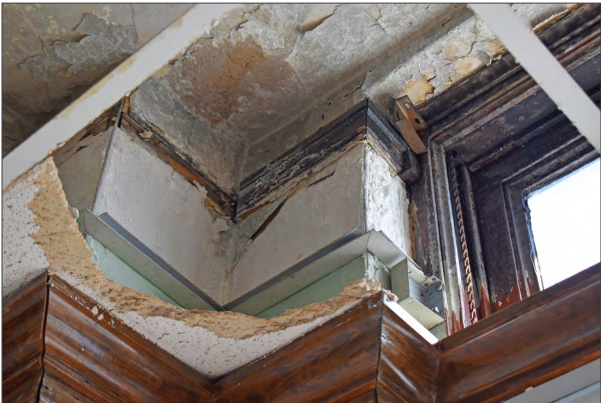
82. Ninth floor, northeast office, older molding
