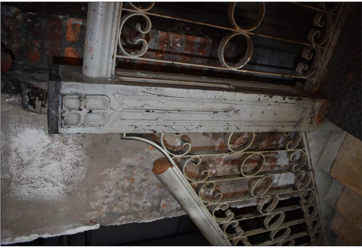
35. First floor, staircase to basement, detail
