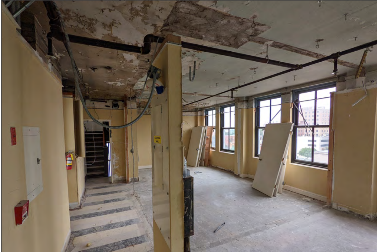
70. Eighth floor, view north towards staircase
