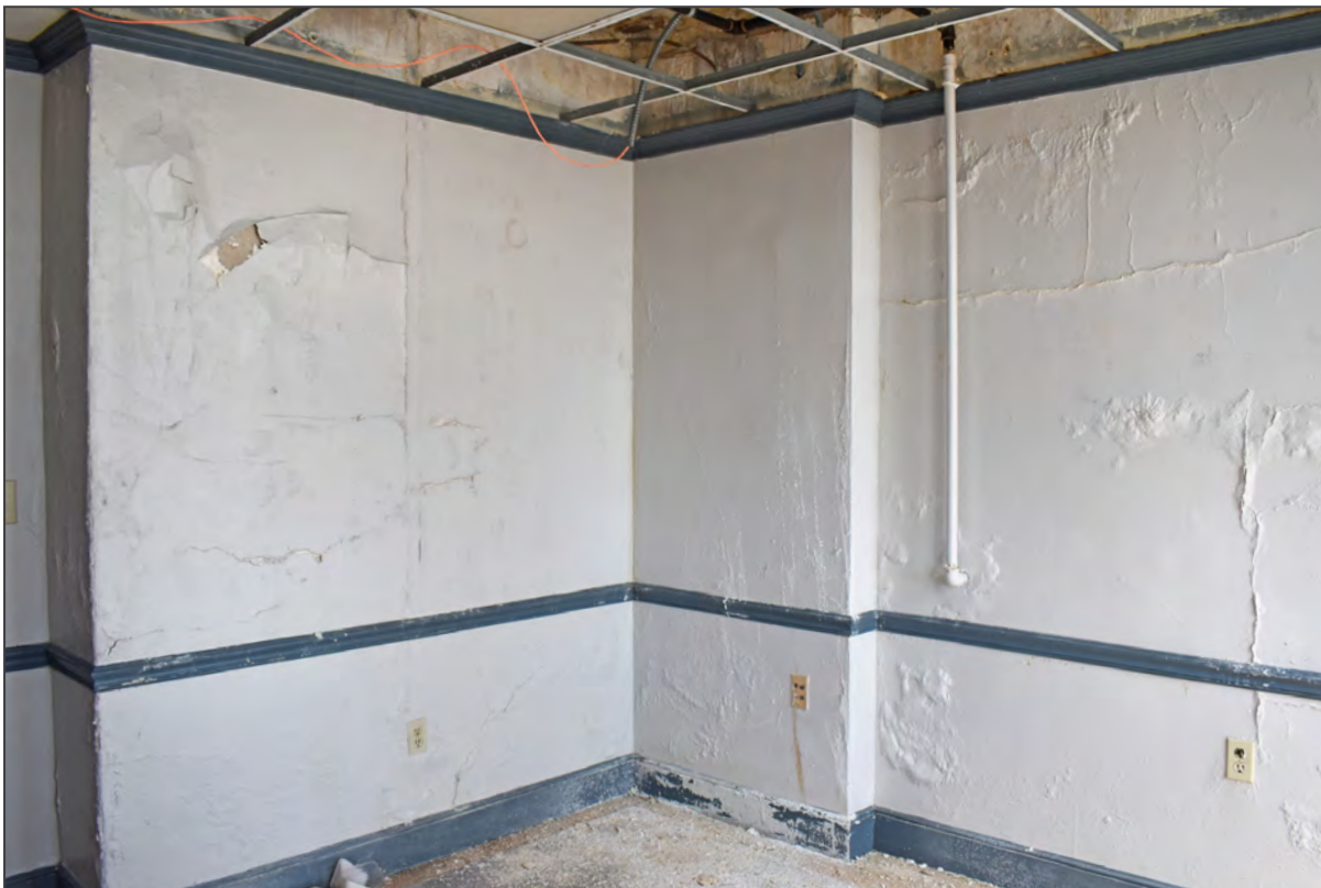
92. Tenth floor, northeast office, view northwest
