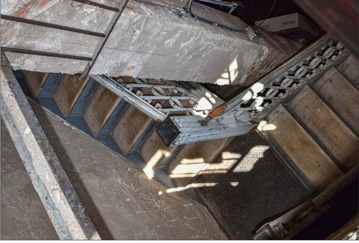
33. First floor, staircase to basement, view northwest
