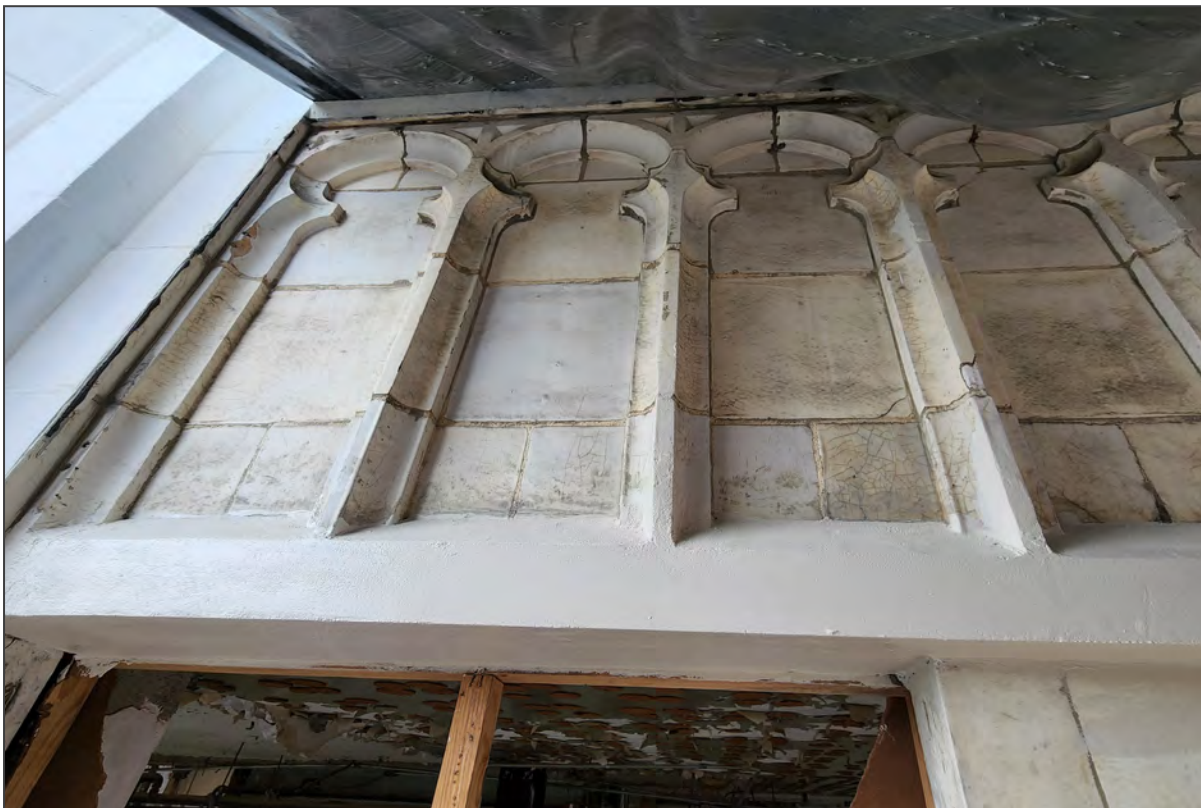
117. Replacement header example, painted.
