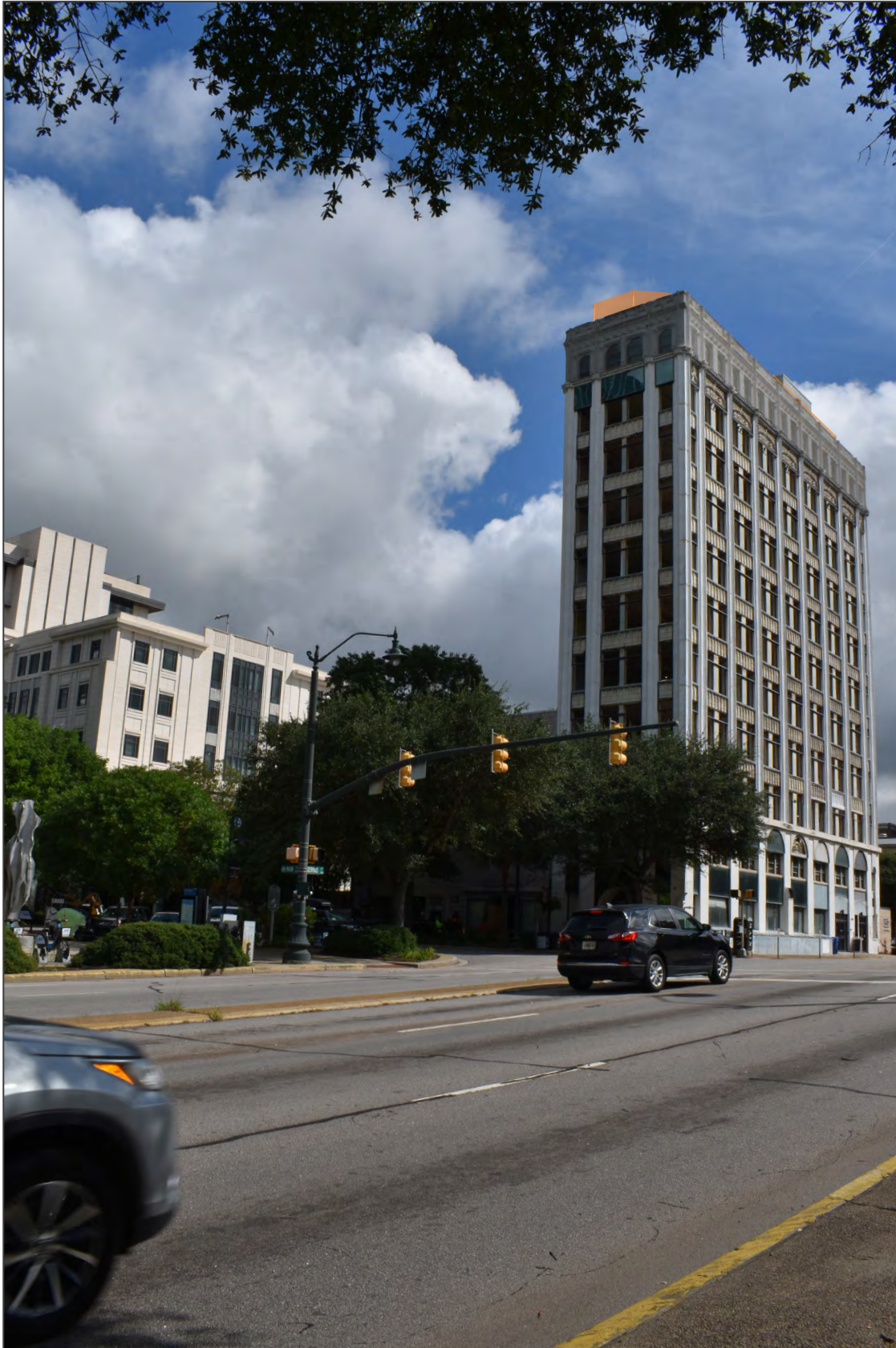
121. Rooftop Bar Mock-up (highlighted in orange), view northeast
