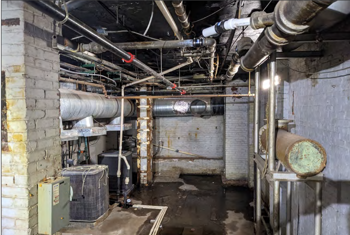
26. Basement, view north
