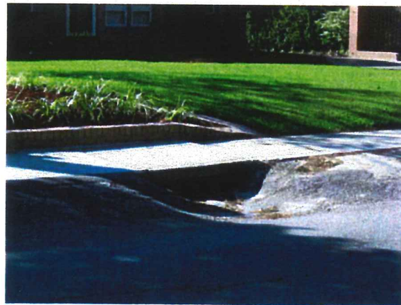
Existing curb and gutter in Greenview
