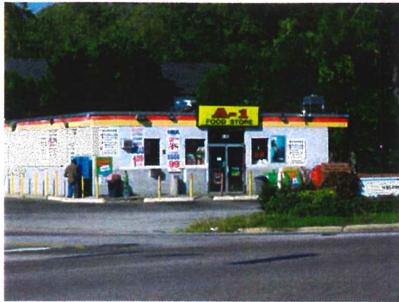
Existing retail at Monticello Road and Duke Avenue
