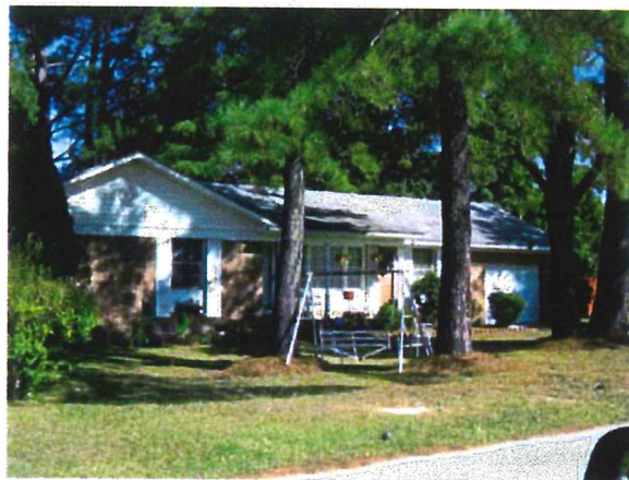
Single-family home in the Fairwold Community
