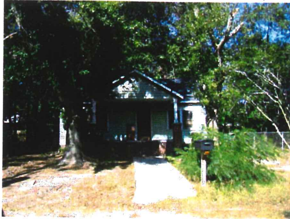
Deteriorating home in Fairwold
