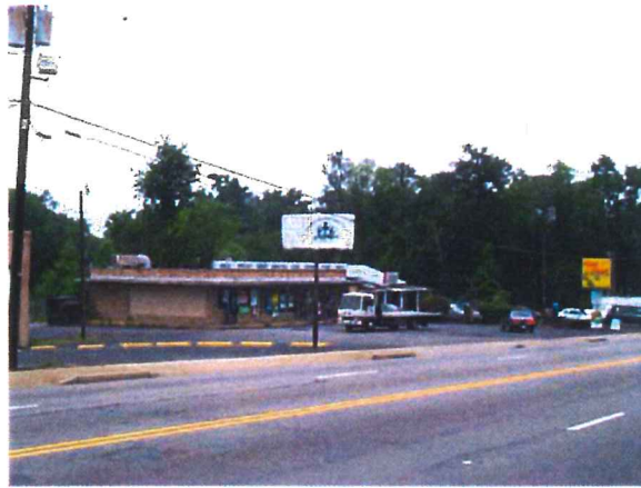
Retail building along Fairfield Road at Winmet Drive
