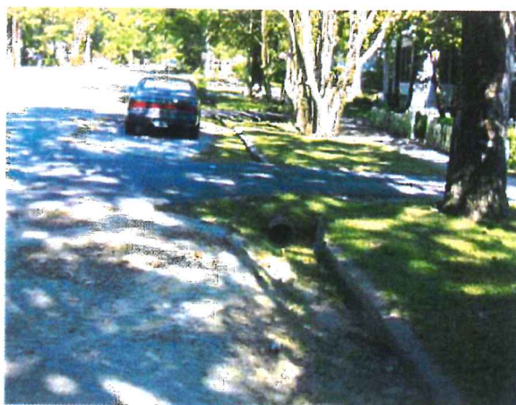
Open storm water ditch in College Place
