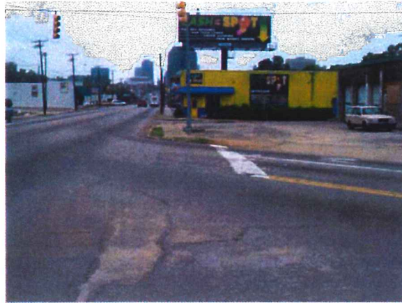
Non-existent crosswalk at N. Main Street and River Drive
