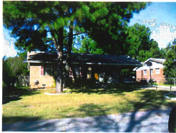
Single-family home in Farrow Terrace
