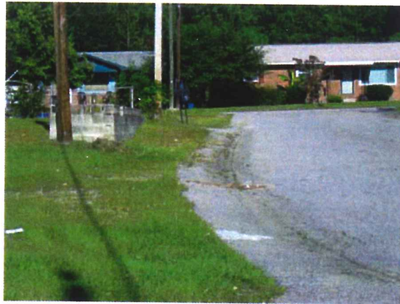
Existing curb and gutter in Farrow Terrace
