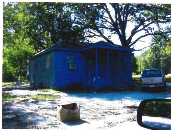
Low quality home in North College Place
