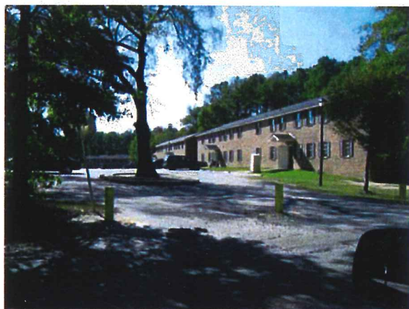
Existing apartment complex in North College Place along Prescott Road
