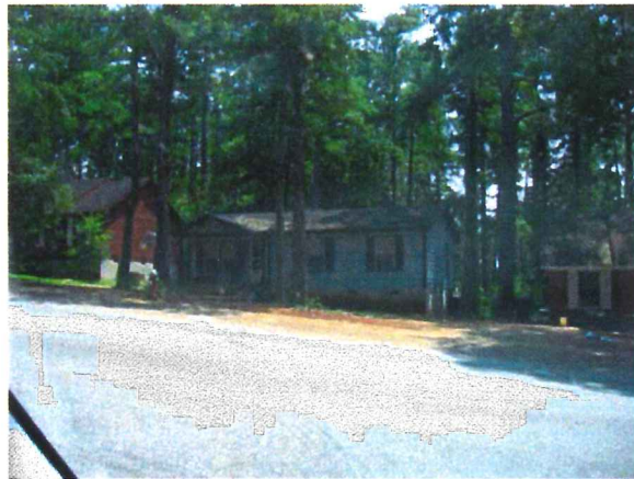
Existing housing inventory on Duke Avenue in Hyatt Park
