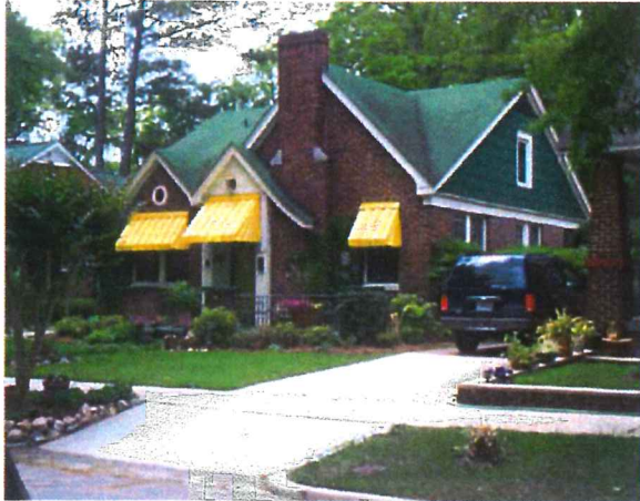
Encourage driveways located within side yard to promote better visual connection to the street
