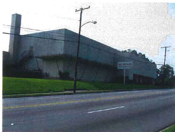
Former Coca-Cola factory
