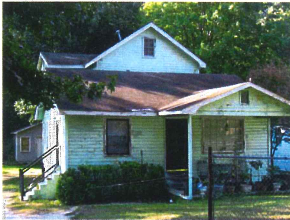
Single-family home that has been converted into multiple residences
