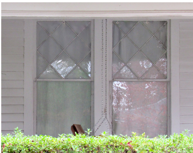
January’s lozenge window, named for its diamond pattern, can be found on a Craftsman Bungalow in Seminary Ridge.
