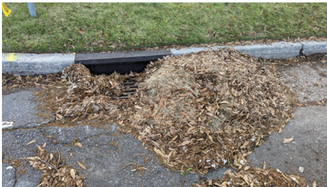
Blocked or overgrown storm drains such as the one pictured above are unable to process heavy rains, and can contribute to surface flooding during storm events.
