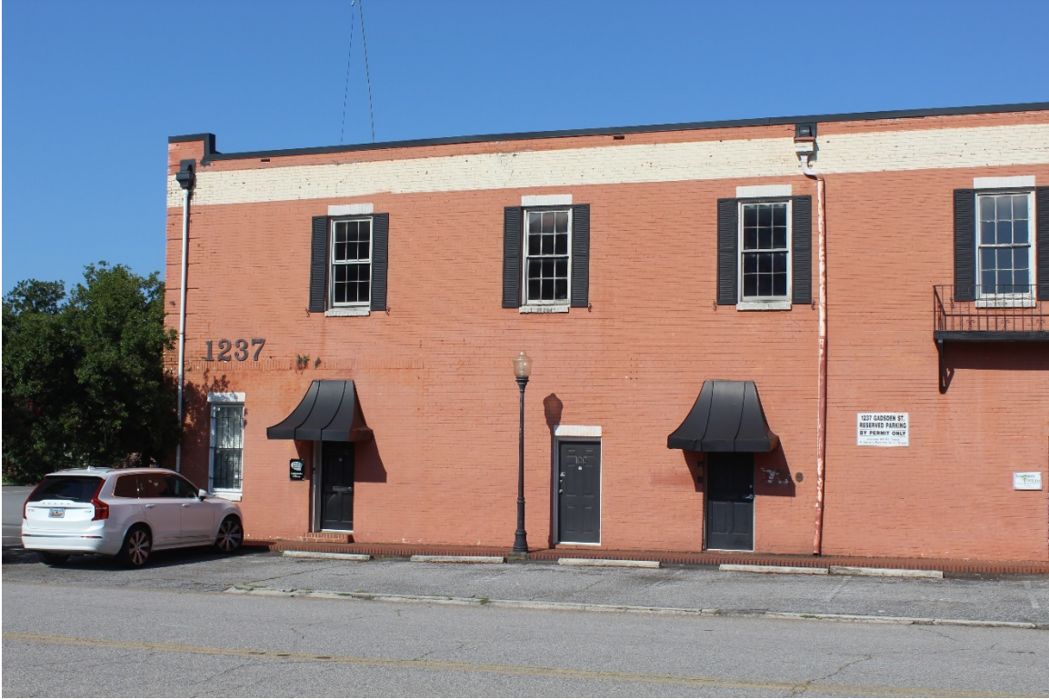
Photo 4 – South end of east façade
