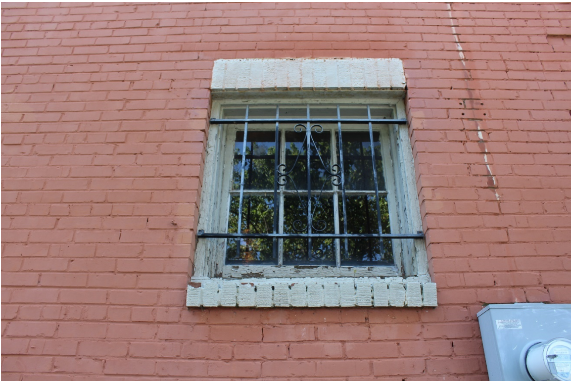
Photo 10 – Original six-light window, north elevation
