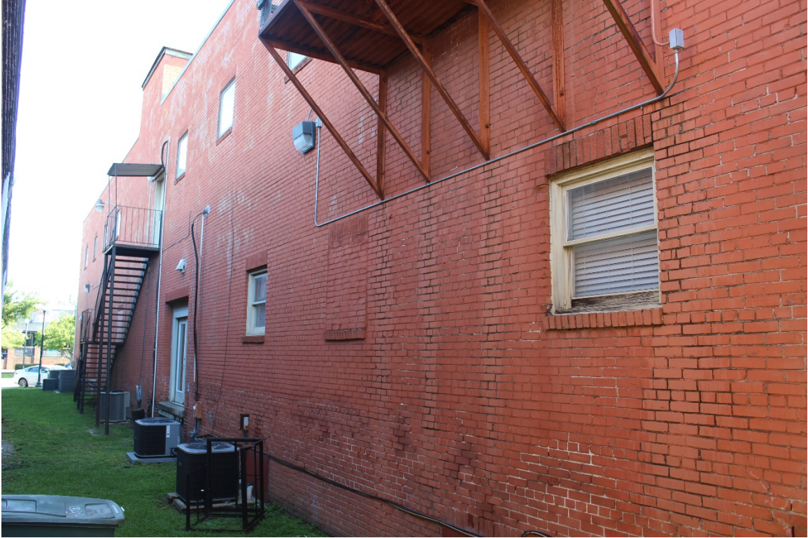
Photo 7 – West elevation, looking north
