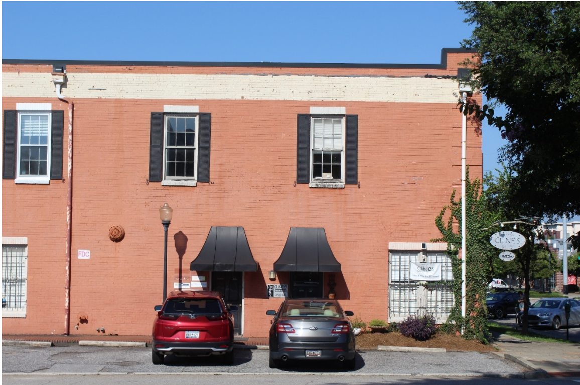
Photo 2 – North end of east façade
