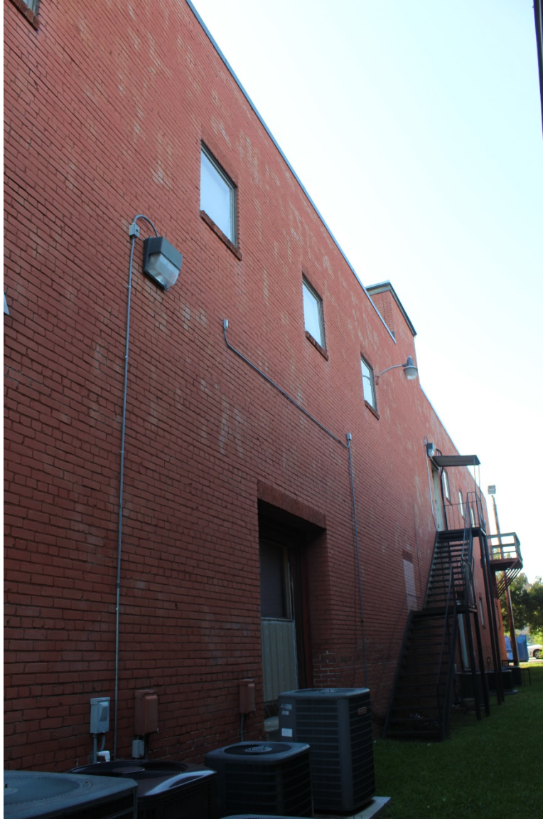
Photo 8 – West elevation with replacement windows and door openings, looking south
