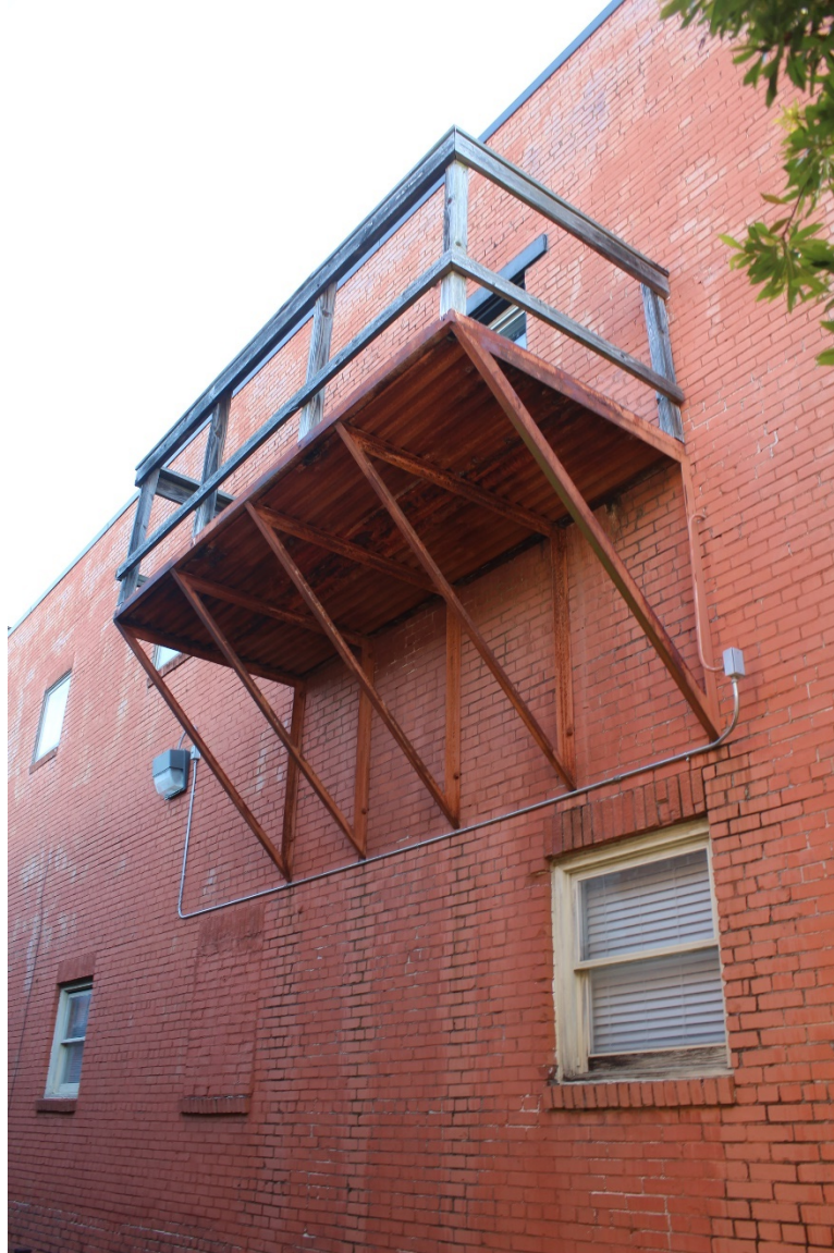
Photo 6 – Replacement and in-filled windows, bracketed metal balcony, west elevation
