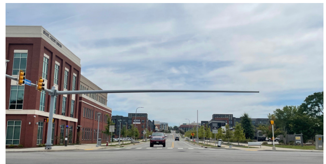
The South Carolina State Credit Union expansion helps define the key intersection of Greene and Huger.
