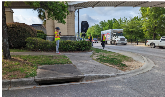
City staff joined SCDOT, consultants, and community stakeholders in a road safety audit of Assembly Street in April. In the above image, auditors investigate the cause for the gap between the sidewalks along Assembly + Wheat streets; surface drainage issues appear to have both eroded and buried the connecting concrete.
