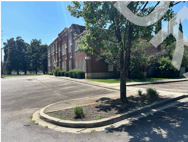
33. Site - parking lot at east elevation to south
