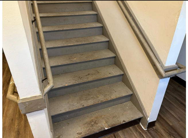
116. Interiors - wood stairs at 2 story wing
