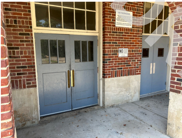
69. Exteriors - older wood entry doors at east elevation
