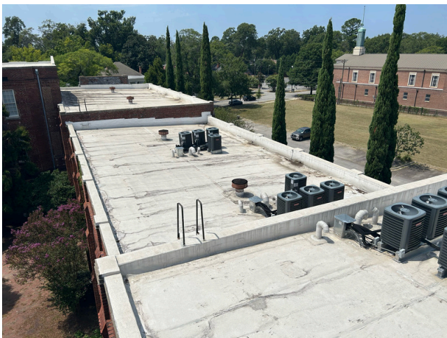
59. Roof - lower roof at rear
