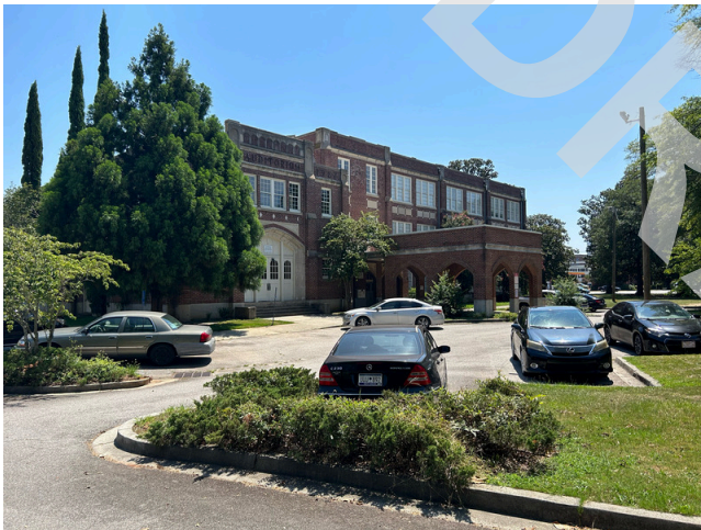
3. Exteriors - overview at west elevation
