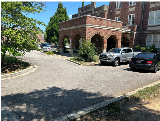
5. Exteriors - overview of main entrance at west elevation
