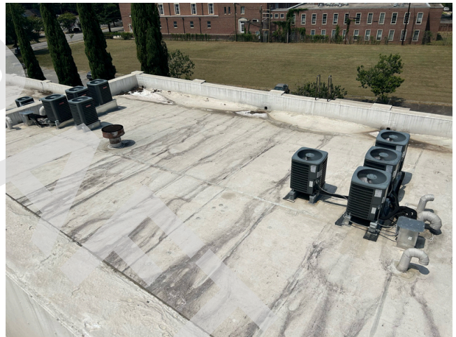
58. Roof - lower roof at rear
