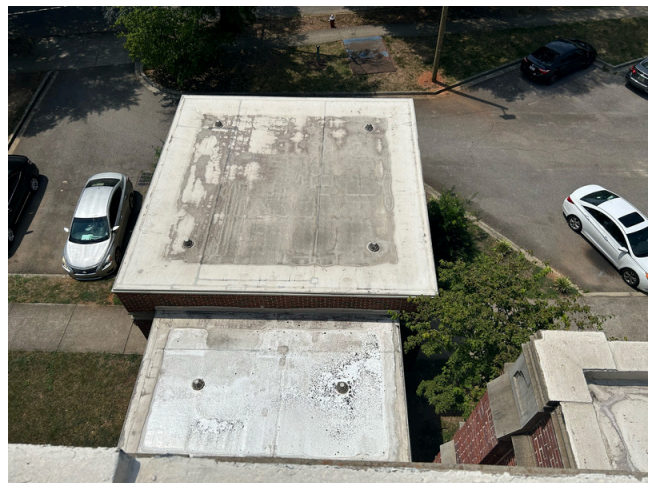
60. Roof - Porte cochere roof system
