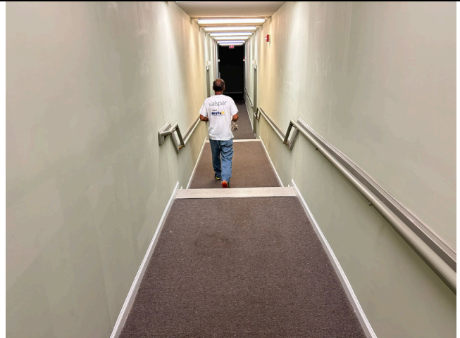
104. Interiors - common corridor to two story wing
