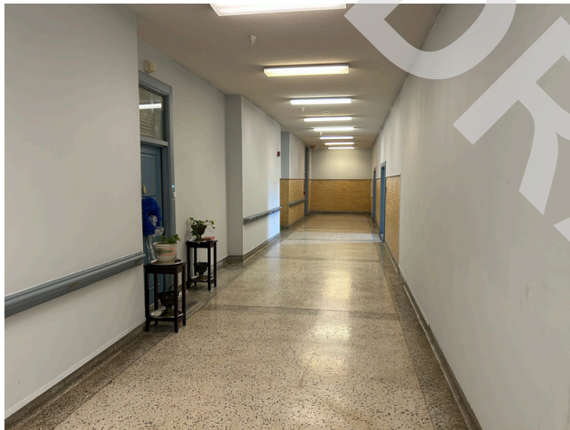
105. Interiors - common tenant corridor
