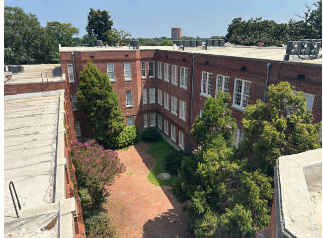
2. exteriors - brick masonry & wood window systems
