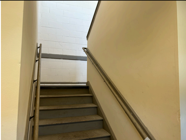
115. Interiors - wood stairs at 2 story wing
