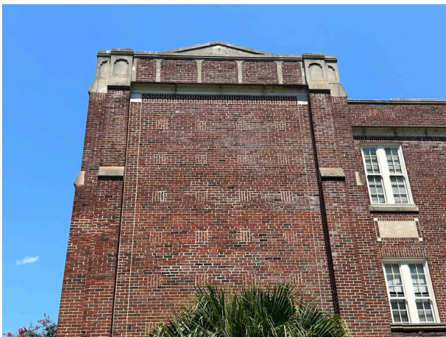
71. Exteriors - typical brick masonry in good condition
