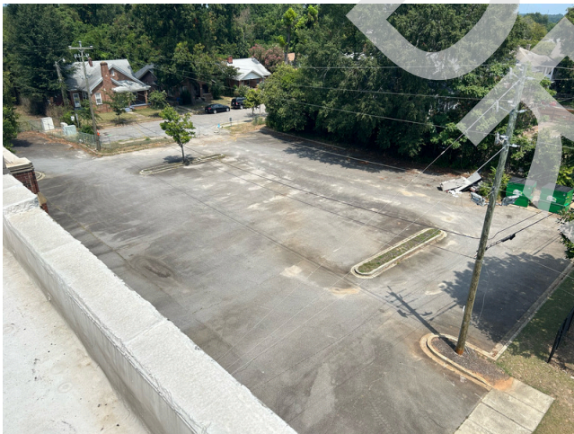
21. Site - asphalt paving at east elevation
