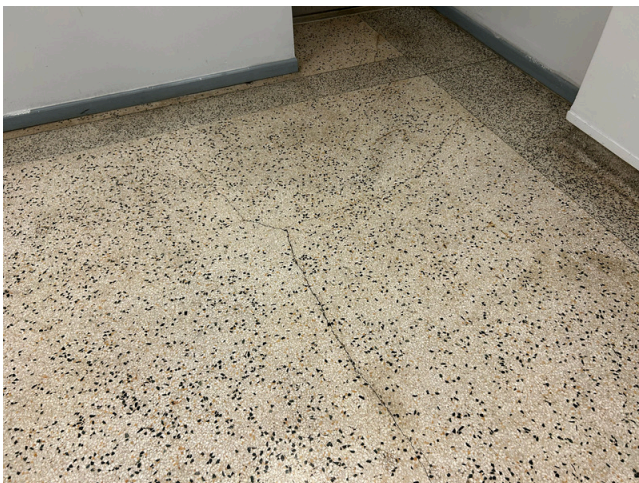
113. Interiors - typical terrazzo condition at common corridor
