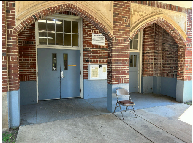
68. Exteriors - main entry at west elevation
