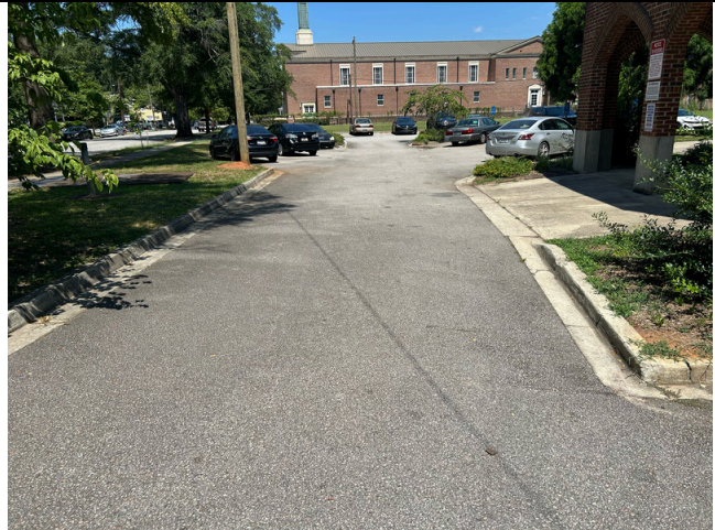
20. Site - asphalt pavement at main entry
