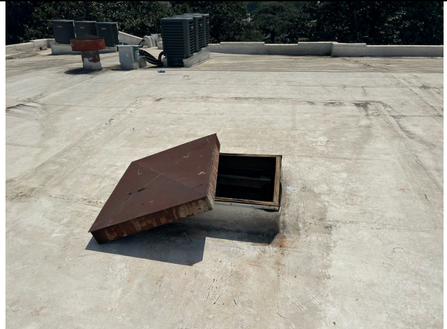
56. Roof - access scuttle at Unit 312
