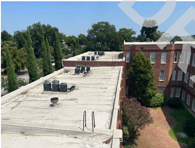
57. Roof - lower roof
