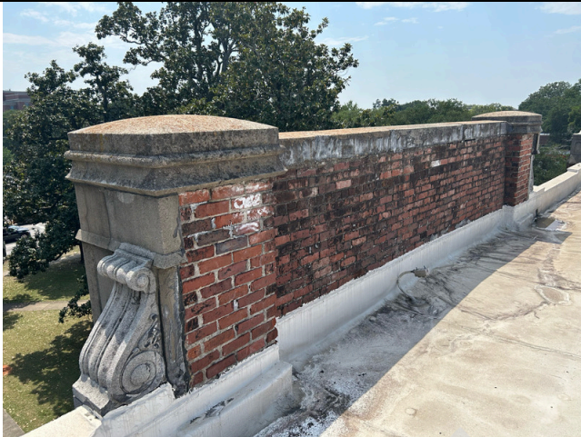
67. Exteriors - brick masonry parapet wall
