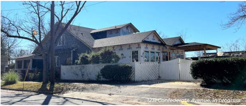
1231 Confederate Avenue, in progress
