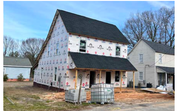
New construction at 507 Denmark Street in progress
