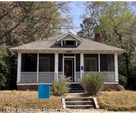
1210 Woodrow Street, before renovations
