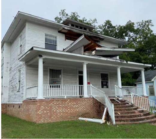
1421 Heidt Street after attempted demolition
