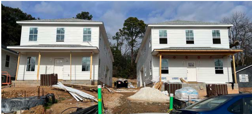
New construction at 2315 & 2317 Greene Street in progress
