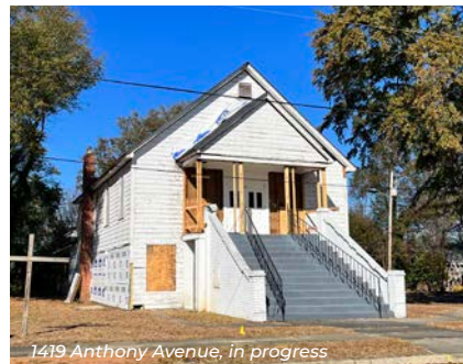
1419 Anthony Avenue, in progress
