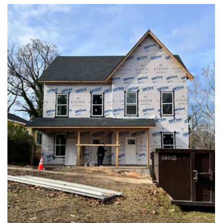
New construction at 817 Heidt Street in progress
