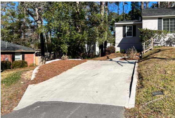
Excess driveway material removed from 3430 Earlewood Drive per D/DRC ruling
