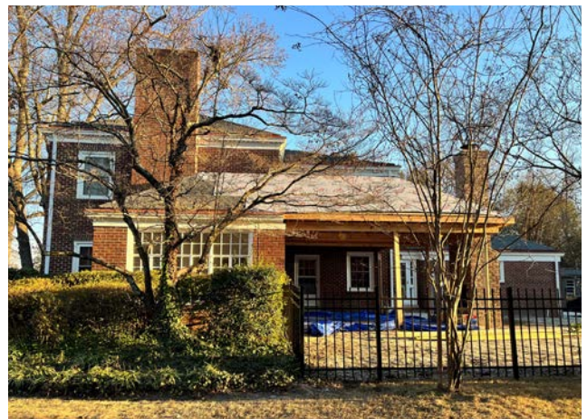
Porch addition at 3200 Amherst Avenue in progress
