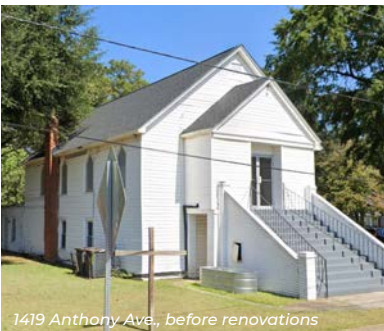
1419 Anthony Ave., before renovations
