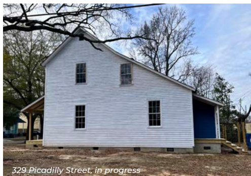
329 Picadilly Street, in progress
