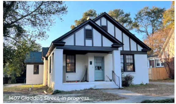
1407 Gladden Street, in progress
