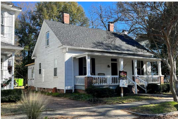
Rear addition at 2304 Lincoln Street in progress
