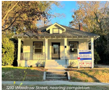
1210 Woodrow Street, nearing completion
