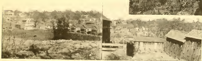
Conditions in Washington Park Area. Dumps, Negro Tenements and Outbuildings
