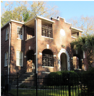
Figure 2.12 Example of projecting porch MMH frontage in Columbia. Upper-story units in the building are accessed by a single, shared entry that leads to a hall or small lobby area.
