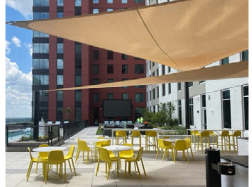
A view of the Standard from the pool deck, taken during the July ribbon cutting celebration.
