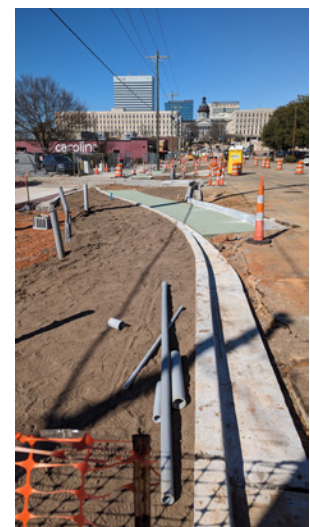
The above photos, taken in February 2024, track the progress of construction. The expansive sidewalks seen on the left will be found on both sides of the street, as will the cycle tracks, emerging in green concrete on the right.
