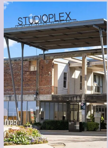
Atlanta offers successful examples of adaptive reuse. StudioPLEX, in Atlanta's Inman Park, offers an example of a redevelopment of a former industrial warehouse into a live-work condominium, where residents operate business out of their urban lofts.
