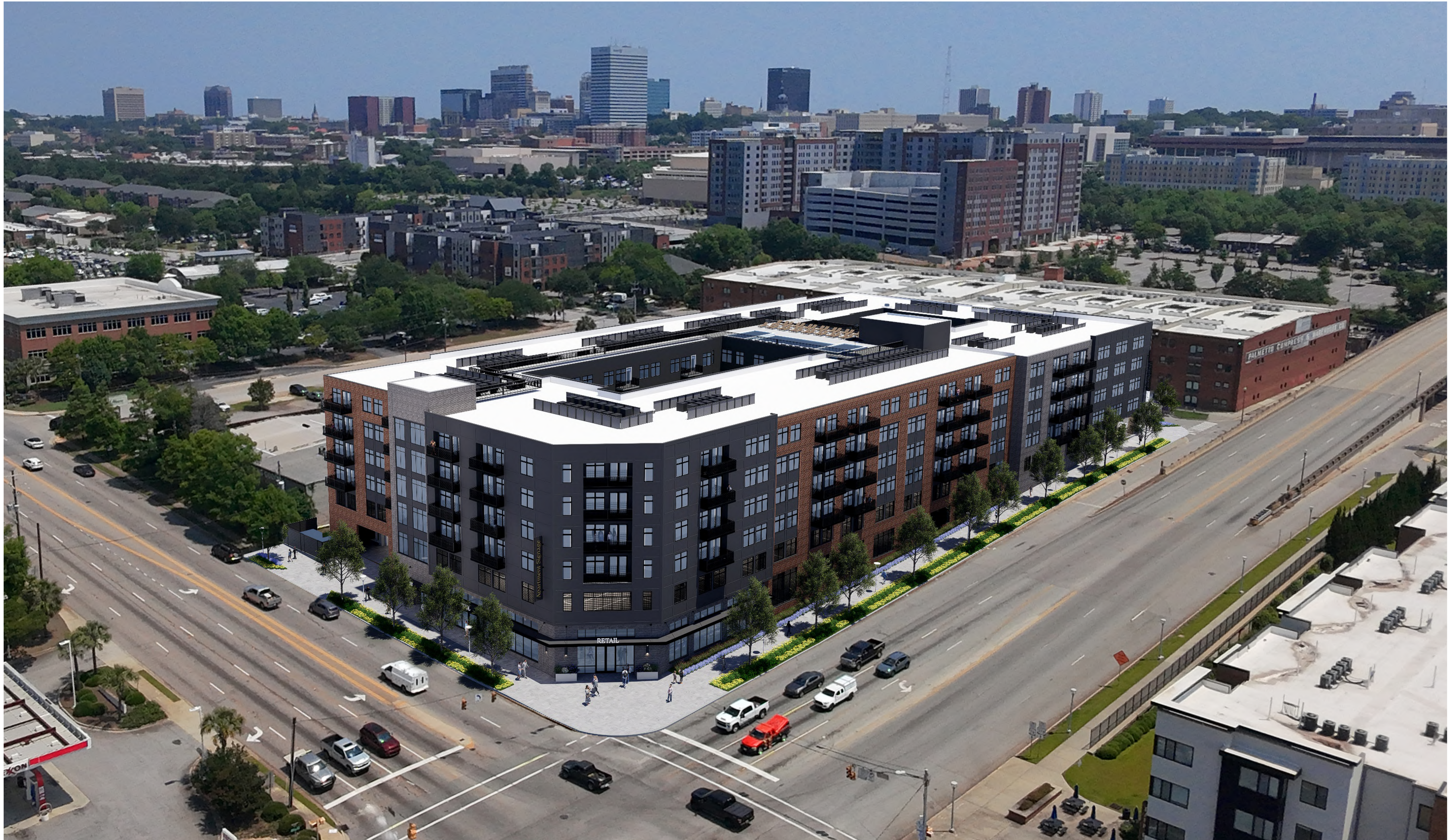
Aerial View from Blossom & Huger Intersection
