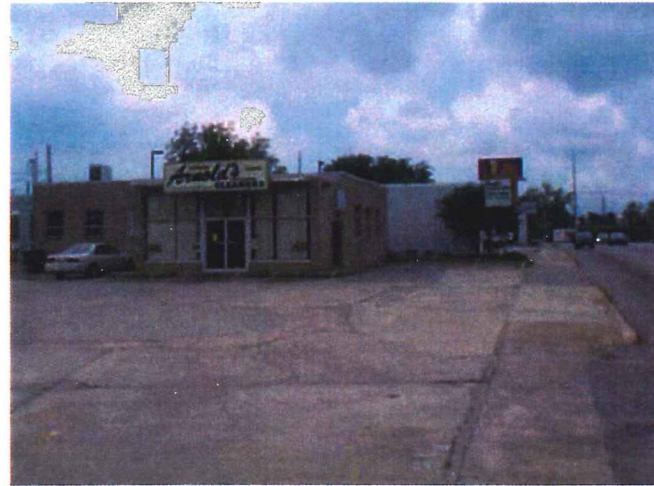
Before - N. Main Street looking north at River Road
