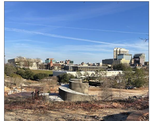
Above: Renovations to Finlay Park during FY 2024-2025.
