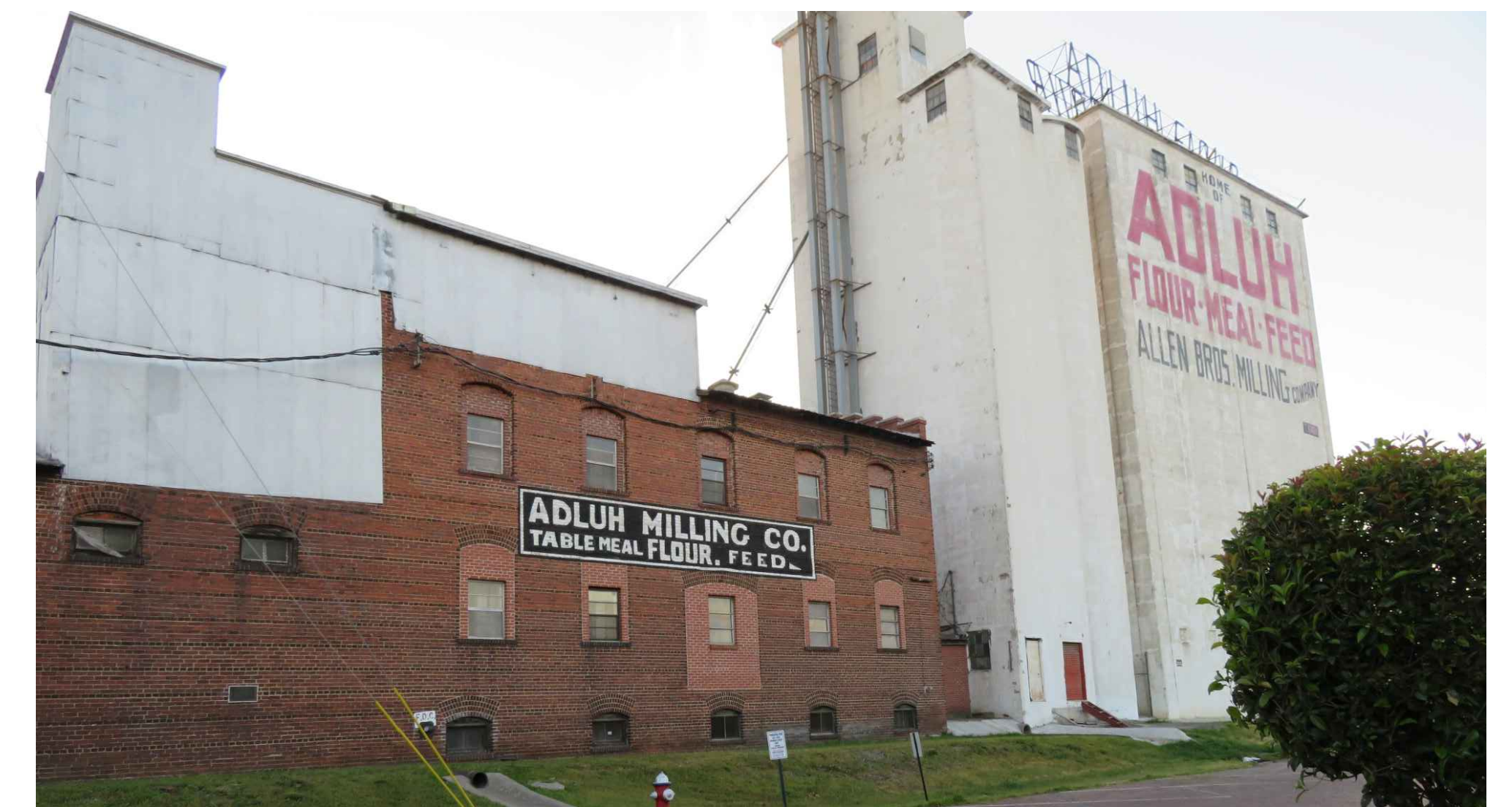
6. VIEW FROM PROPERTY. LOOKING TOWARDS ADLUH MILL
