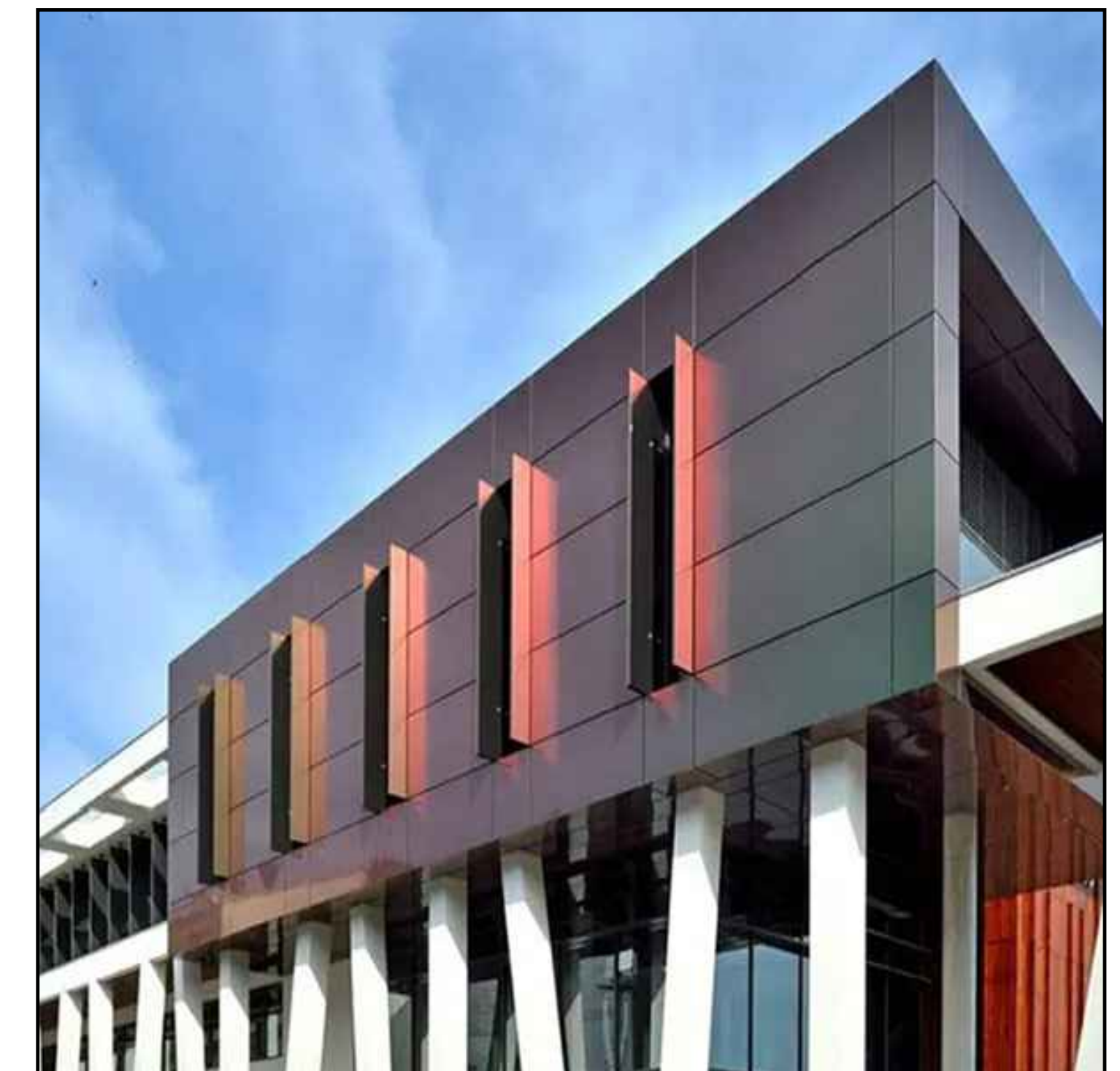
CENTRIC EXTERIOR PANELS: METAL COMPOSITE PANEL WITH PRISMATIC FINISH
