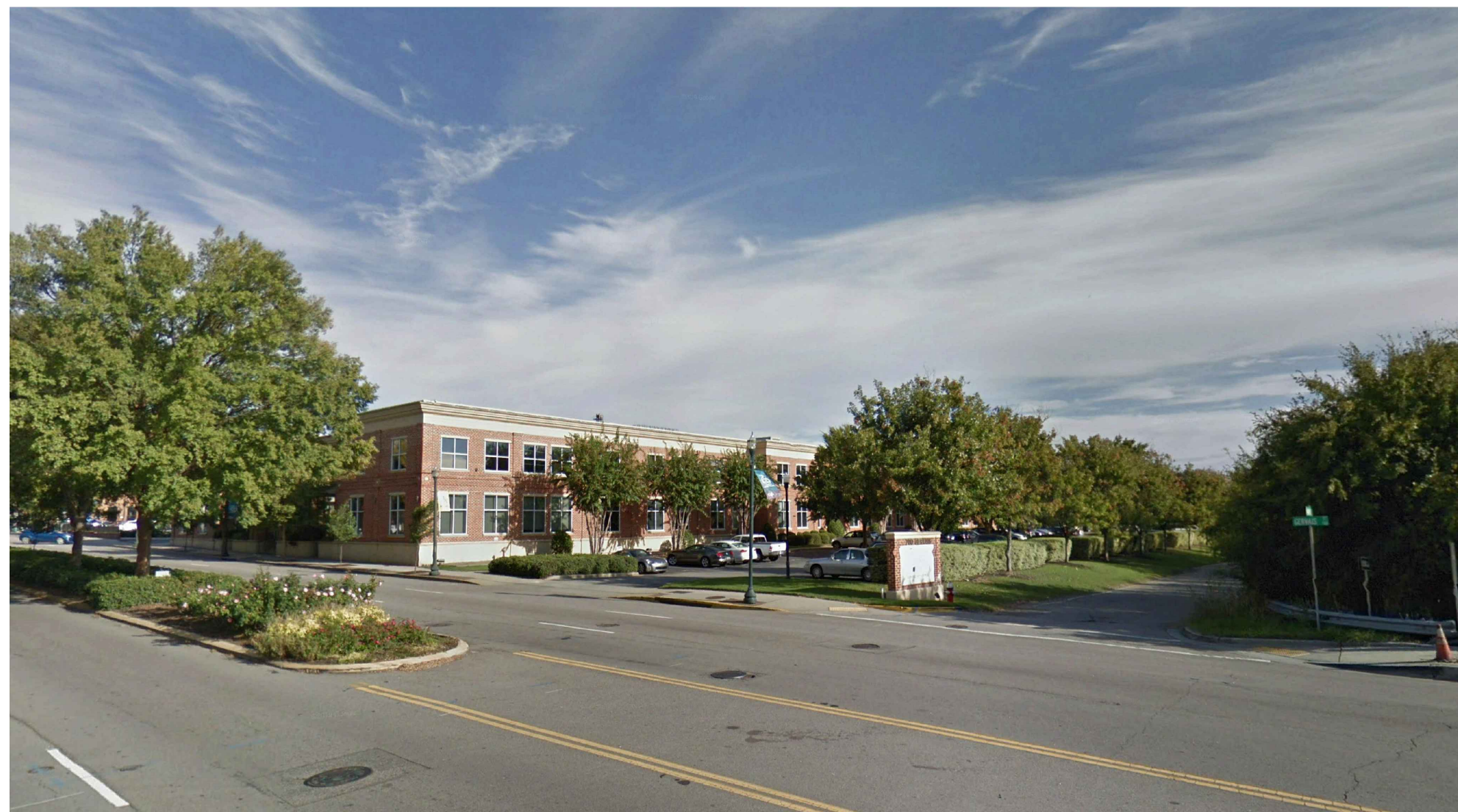
1. VIEW FROM GERVAIS ST. AND WAYNE ST. LOOKING TOWARDS EXISTING OFFICE BUILDING
