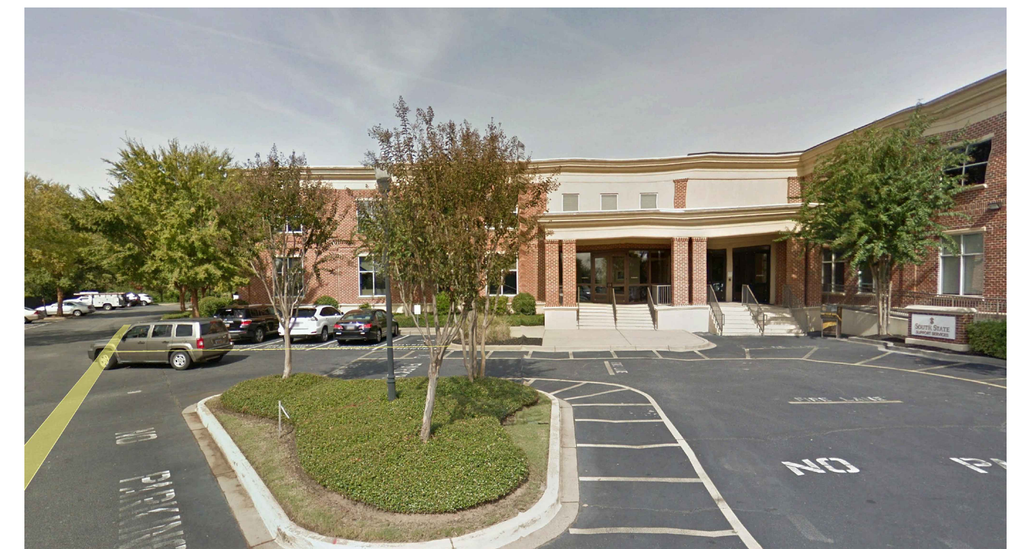
9. VIEW FROM REAR OF PROPERTY. LOOKING TOWARDS EXISTING OFFICE BUILDING
